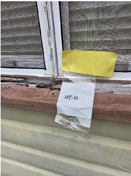
Sample 123-10 Typical Exterior Caulking Sample
