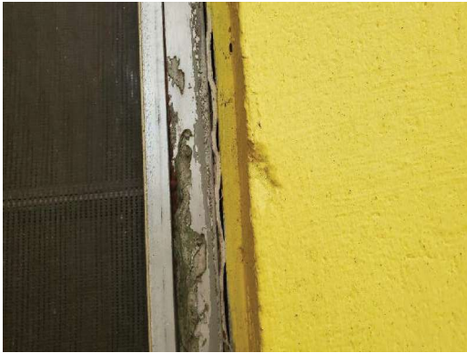
1941-2 Caulk/White Typical Exterior Windows
