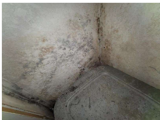
Interior Northwest Bedroom Closet Drywall walls, plastic storage bin Visible water damage Visible microbial growth
