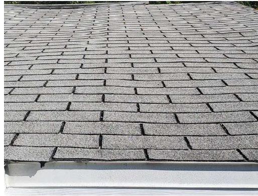
1941-1 Asphalt Shingle/Tar Typical Exterior Roof
