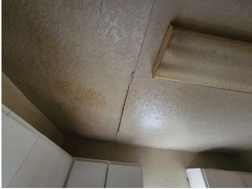
Interior Kitchen Drywall ceiling Visible water damage (cracking)
