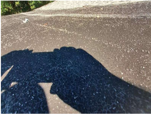
1941-6 Rolled Roofing Typical Exterior Porch
