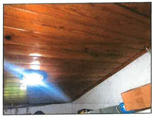
(2) We noted a crack on the ceiling in the front room of the salon, this crack is where the addition was added to the existing building, settlement cracks are common at the joining points. We recommend further review and repair or replace by a qualified person if the crack increases in size.
