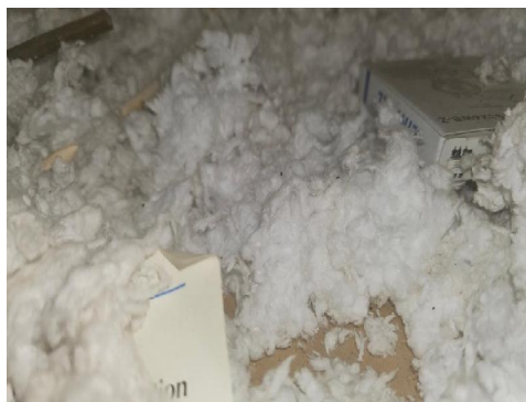
2190-3 Insulation Typical Interior
