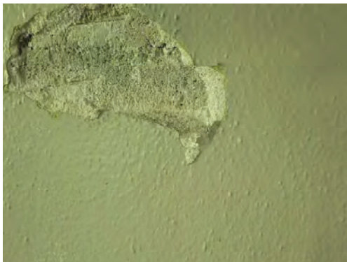
1656-3 Plaster/Rough Coat Typical Interior Walls
