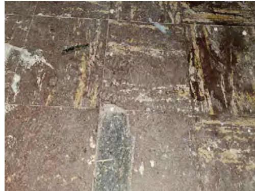
1656-2 9"x9" Floor Tile/Brown (4% Chrysotile) Mastic Interior Bedroom (Appx 250 sq ft)
