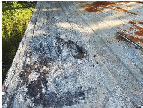
1821-4 Roof Coating/Silver (2% Chrysotile) Tar Typical Exterior Roof
