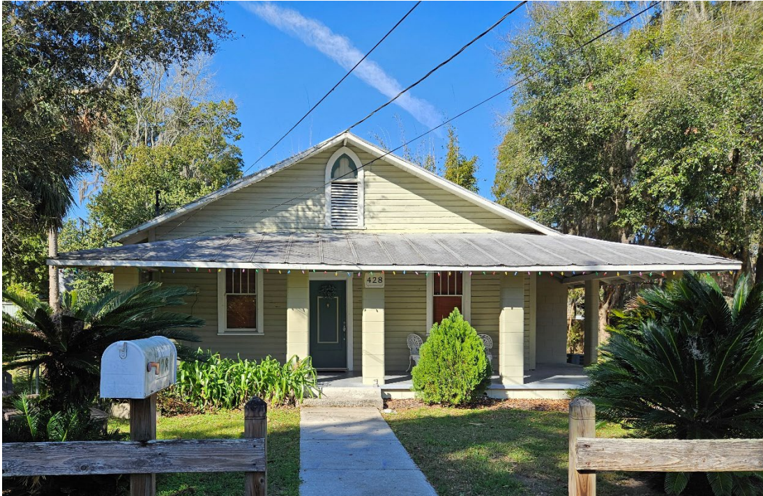
428 NE 7 th Terr Before Photos
