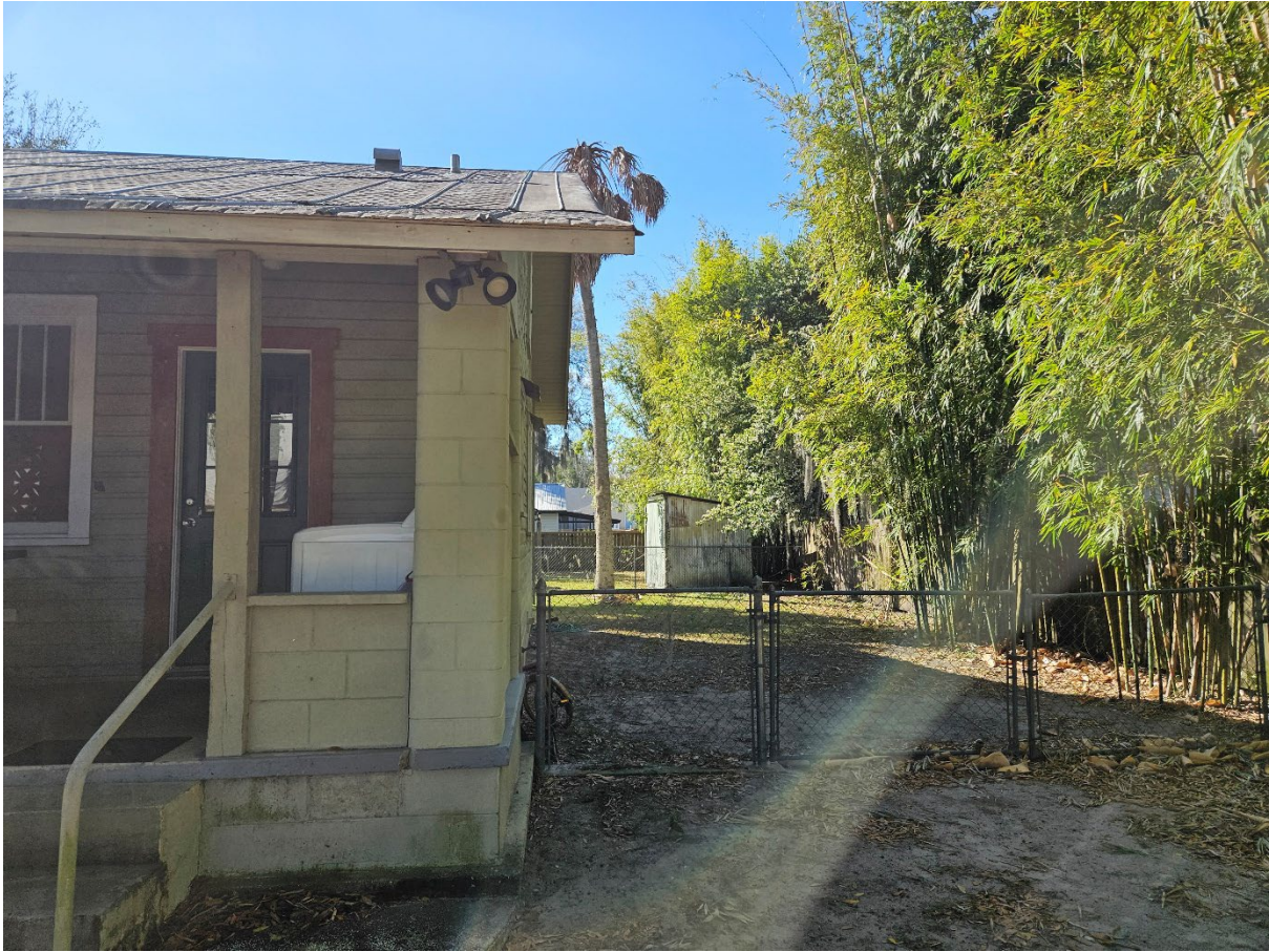
428 NE 7 th Terr Before Photos
