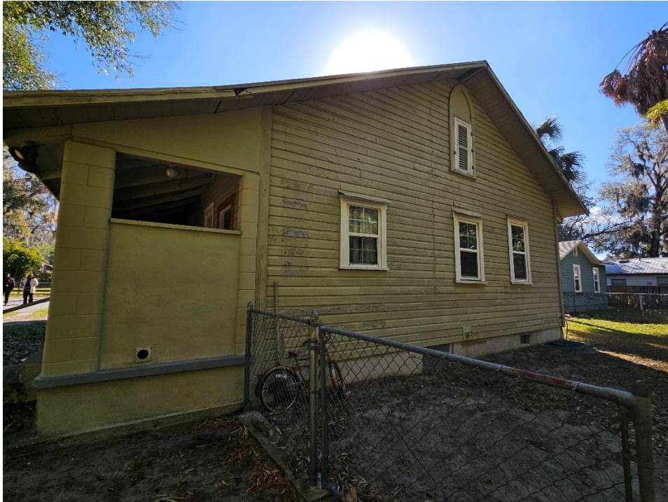
428 NE 7 th Terr Before Photos
