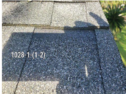
1028-1 Asphalt Shingle/Black, Tar/Black Typical Exterior Roof
