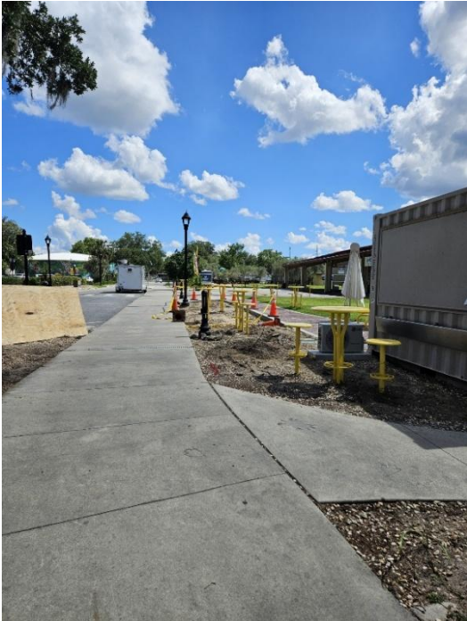
DOWNTOWN MARKET - IMPROVEMENTS IN-PROGRESS
