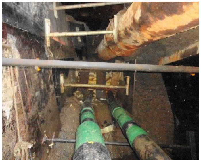
345kV Underground Transmission Line
