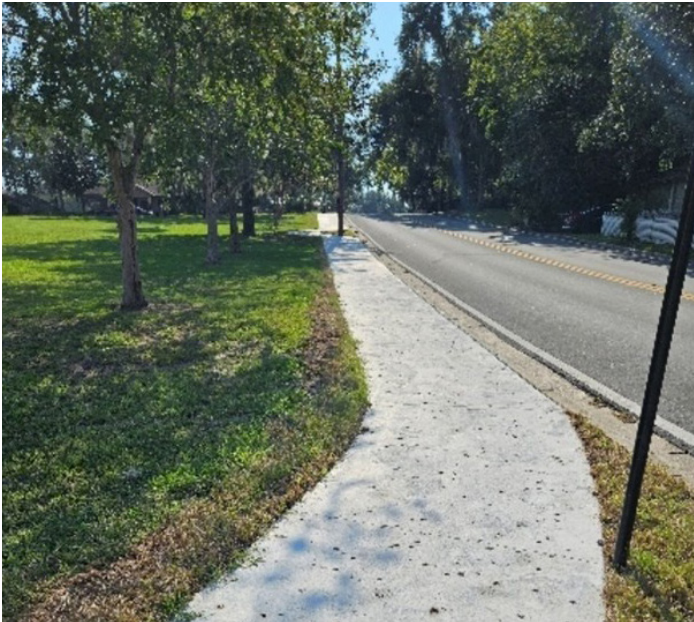
Sidewalk improvements along NE Third St.
