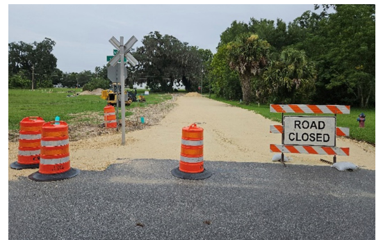
Road construction in progress
