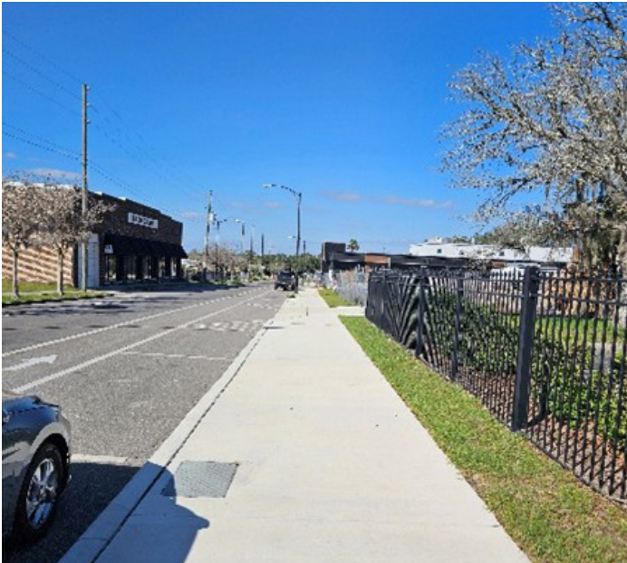
Sidewalk improvements along NE First Ave.
