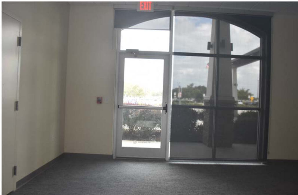
Interior view of typical office.
