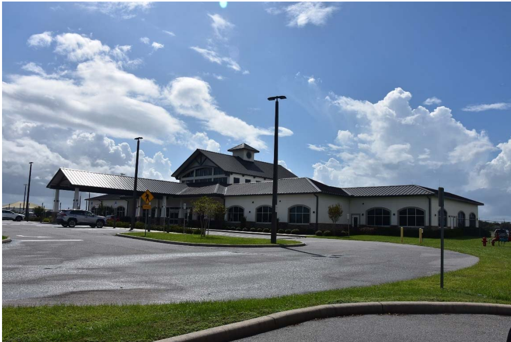
View of east and north elevations.
