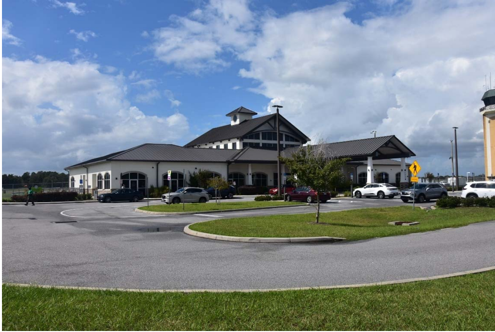
View of east and south elevations.
