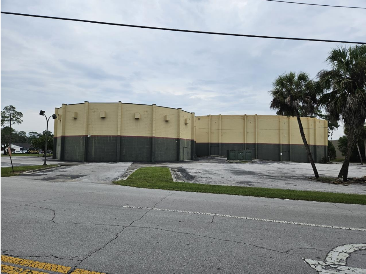
Image 2. View of the building from NE 7 th Street.
