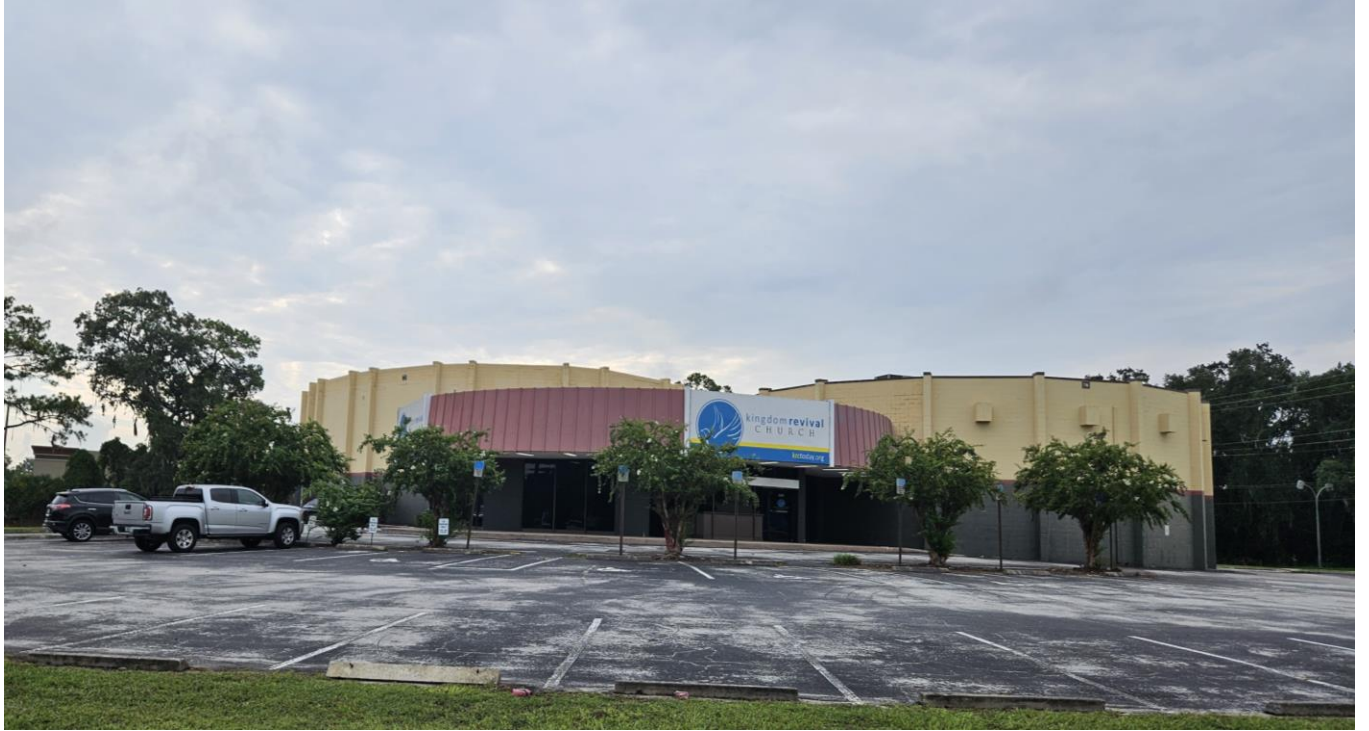
Image 1. View of the building from E. Silver Springs Boulevard
