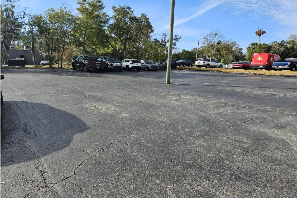
Image 7. Existing condition of parking lot.
