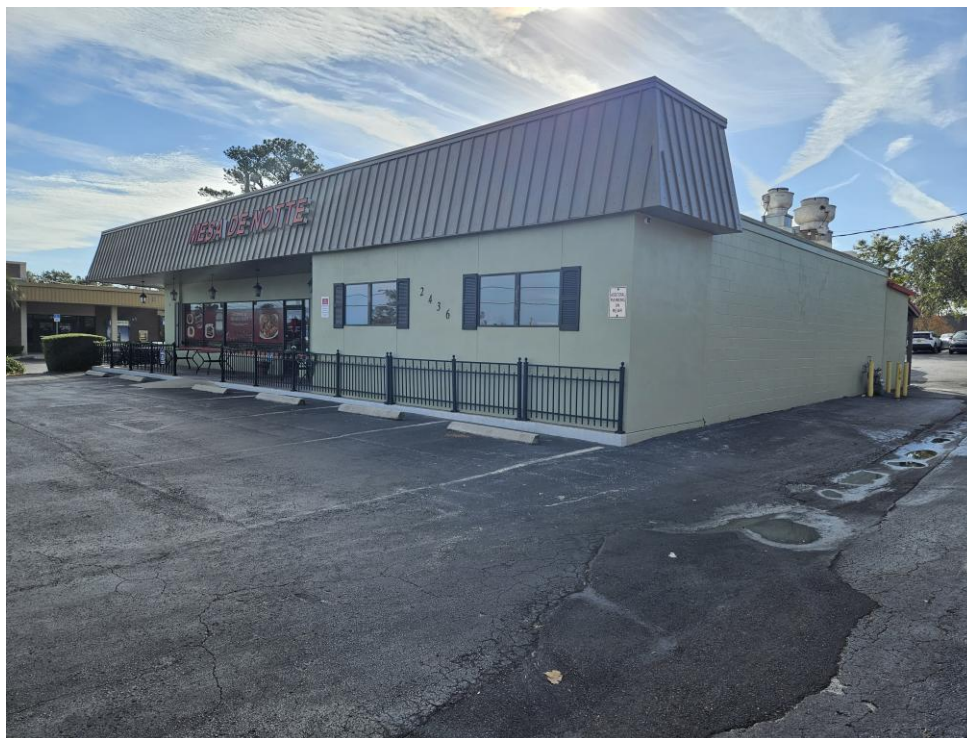
Image 2- Existing conditions -side view
