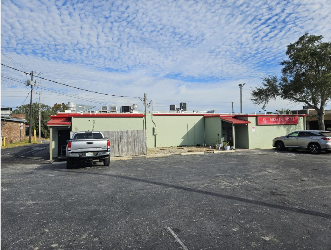
Image 6 – Existing condition of parking lot
