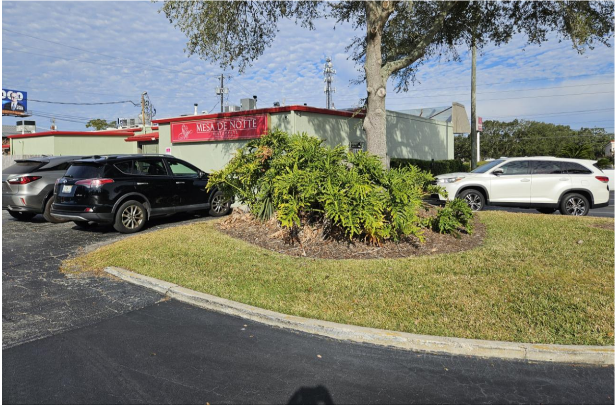
Image 3 – Existing condition – Rear entrance
