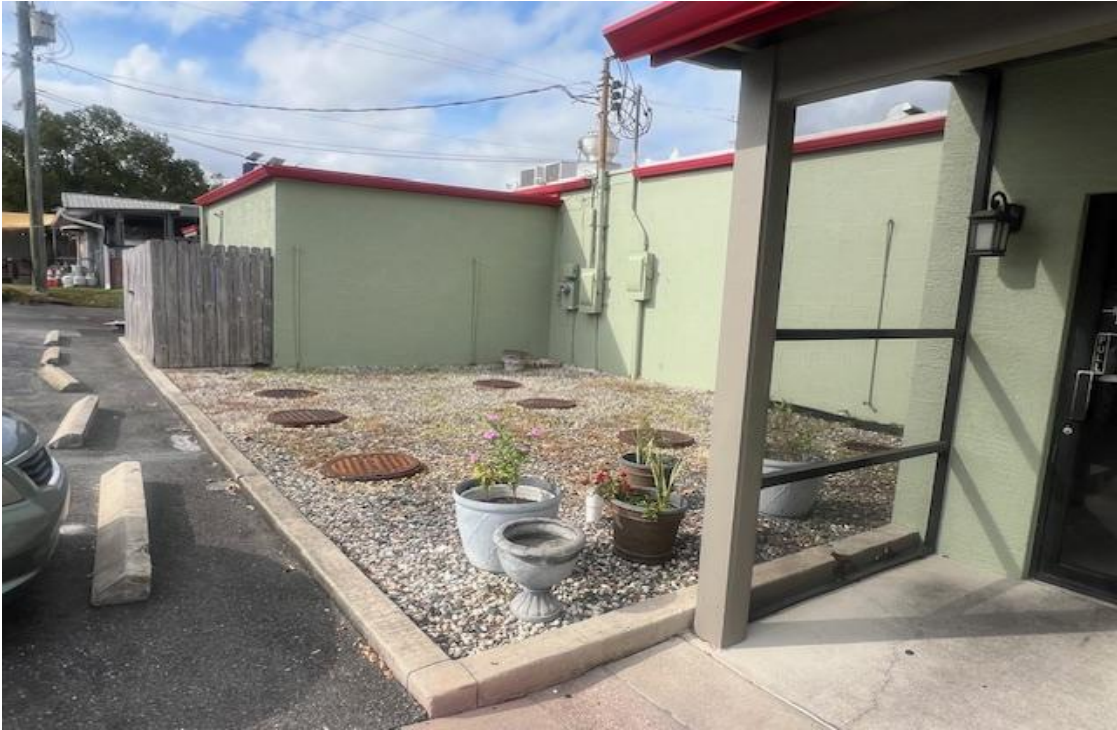
Image 5 -Existing condition – Rear view and entrance
