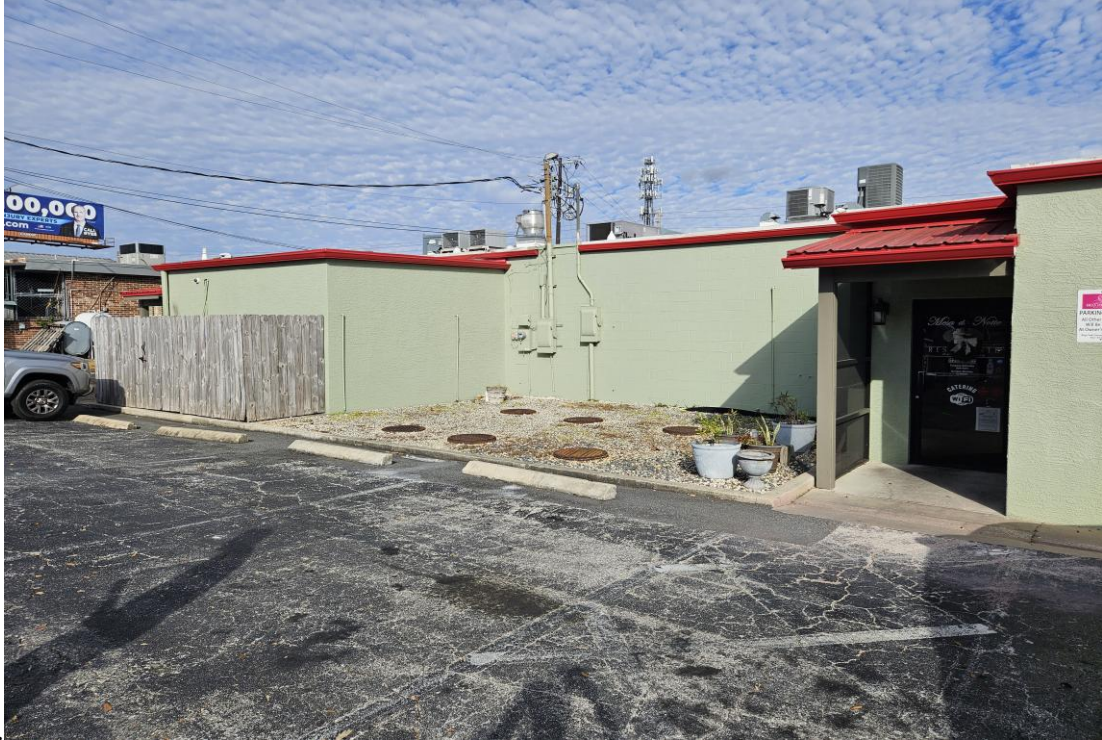
Image 4 – Existing Condition – Rear view and entrance
