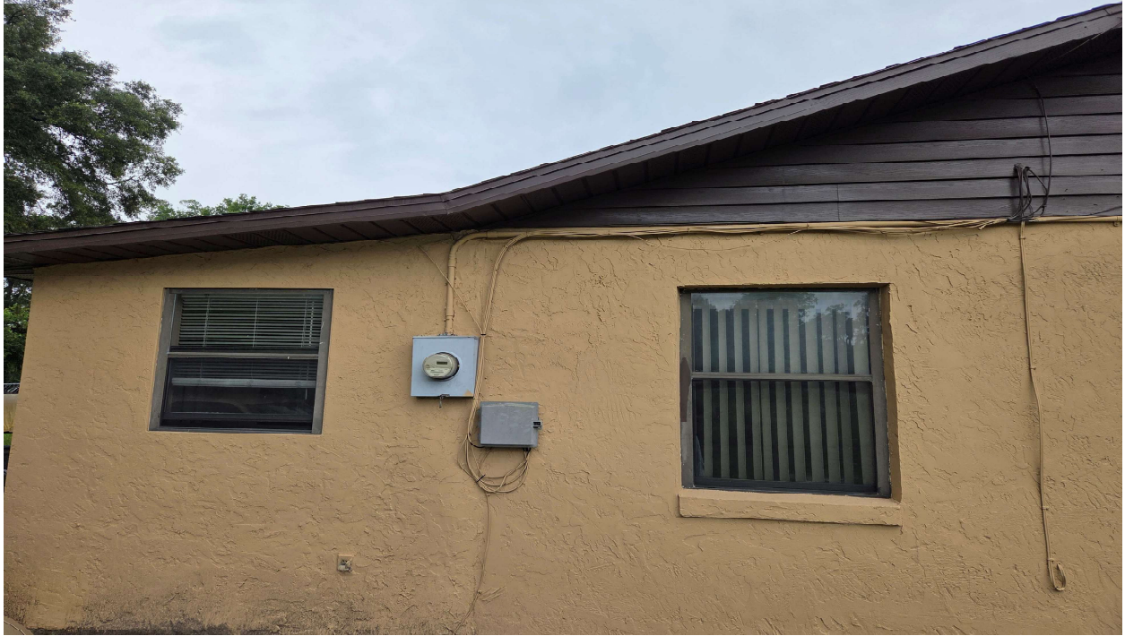
Image 2- Existing window conditions
