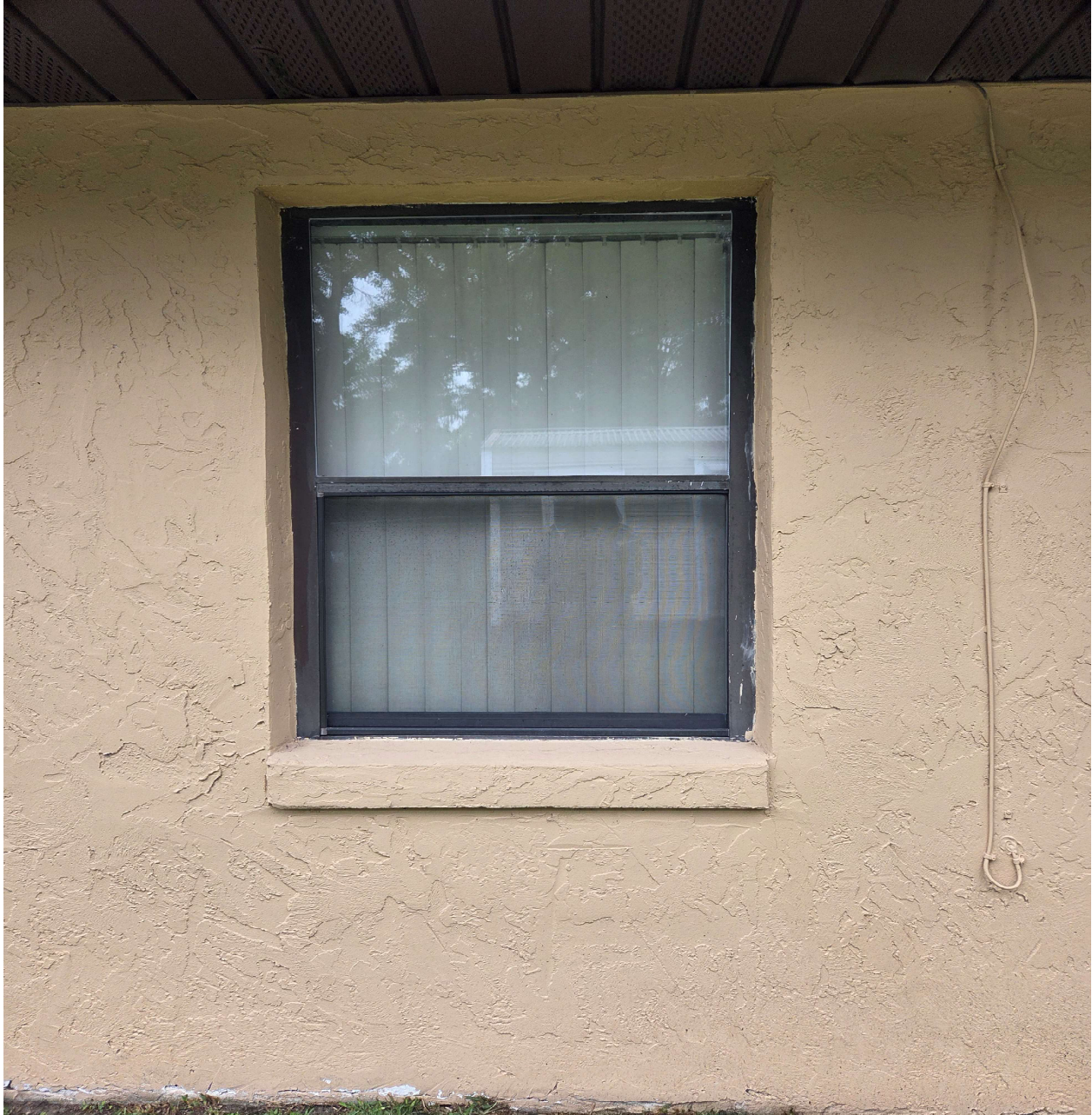
Image 4- Existing window conditions
