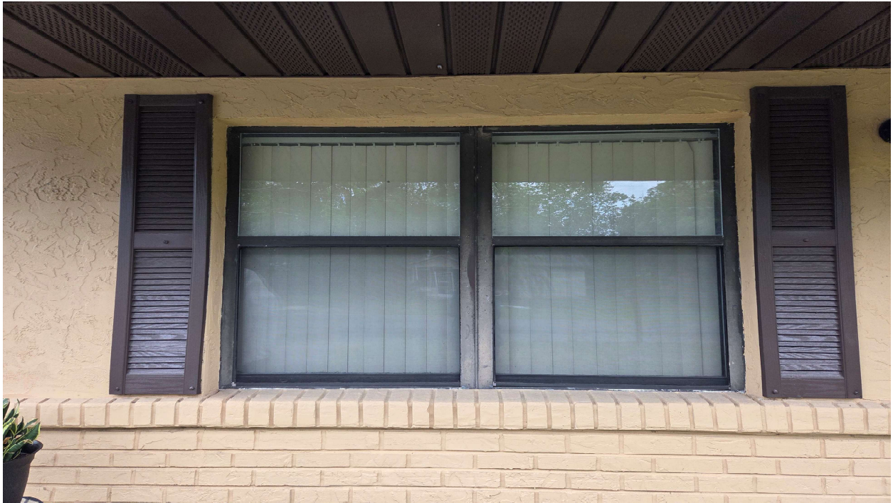
Image 3- Existing window conditions
