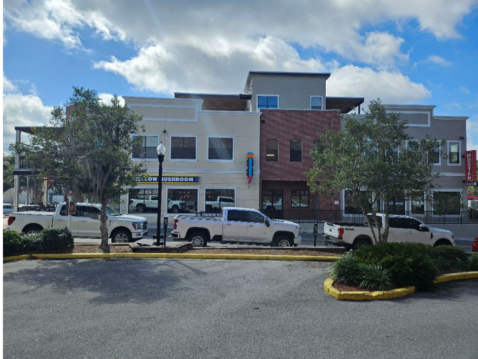
Figure #. North elevation after completion.
