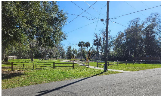
Figure# After – Completed project.
