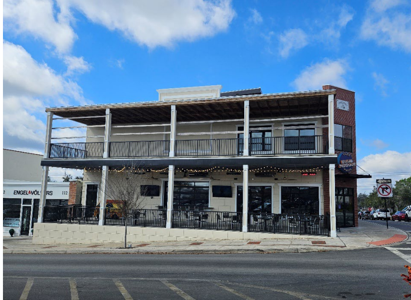
Figure #. East elevation after completion.
