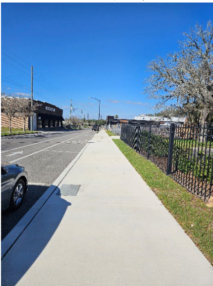
Figure# Sidewalk improvements along NE 1 st Avenue.
