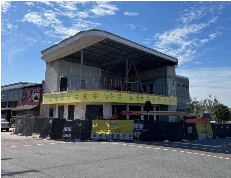
Figure # Construction - in progress.
