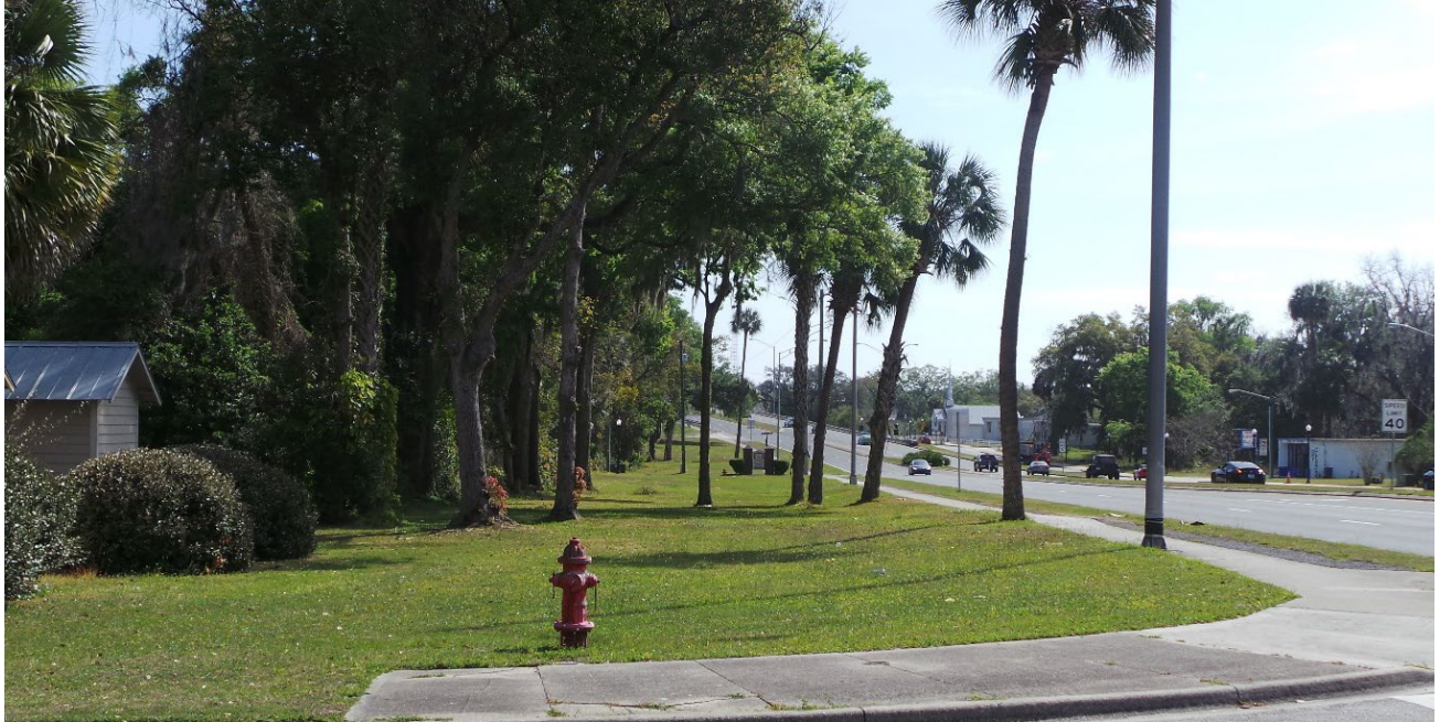
Figure # Site conditions before improvements, looking east along West Silver Springs Boulevard.
