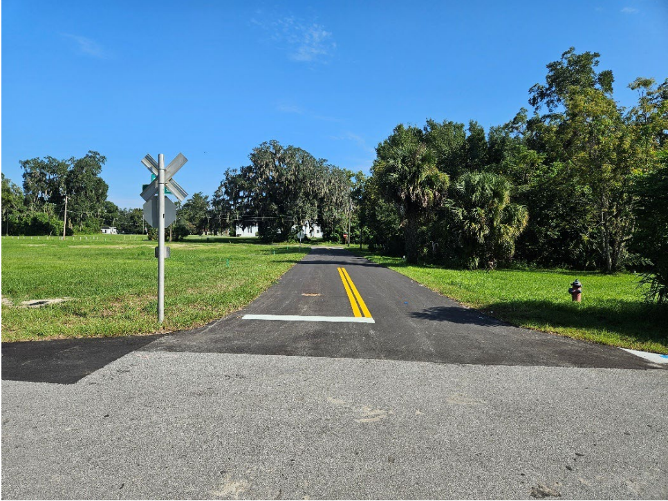
Figure # Newly constructed road.
