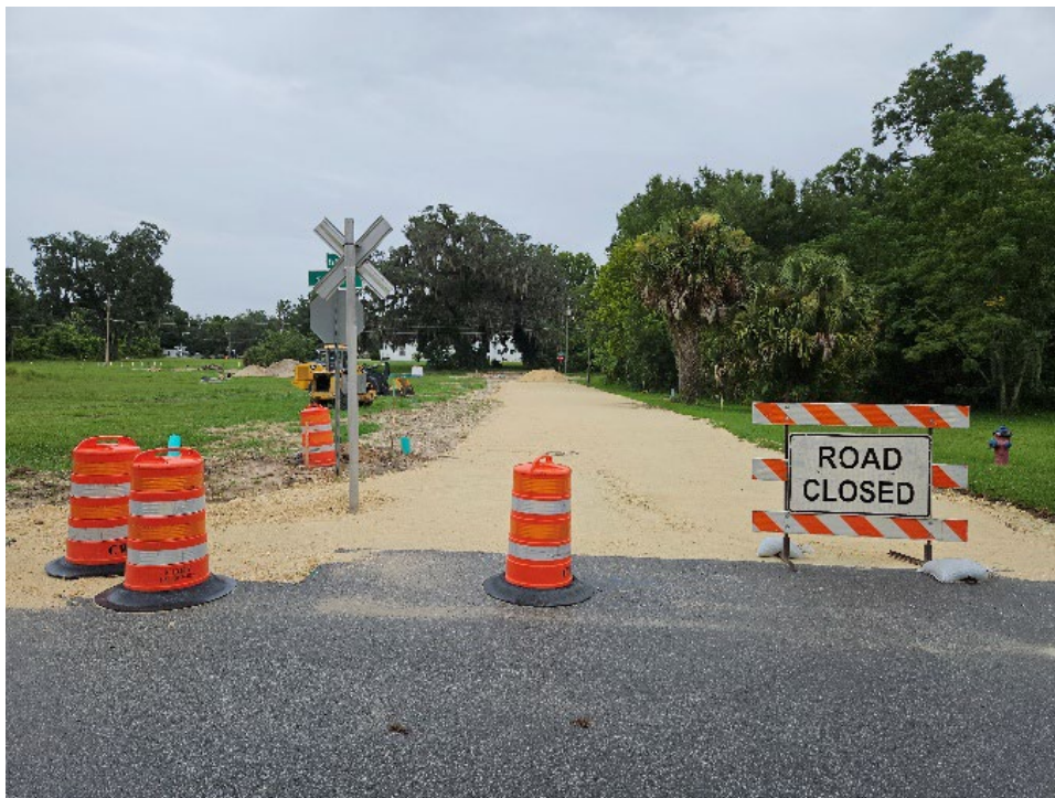
Figure # Road construction in progress.
