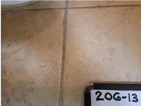
206-13 Grout Typical Interior Hall Bathroom Flooring
