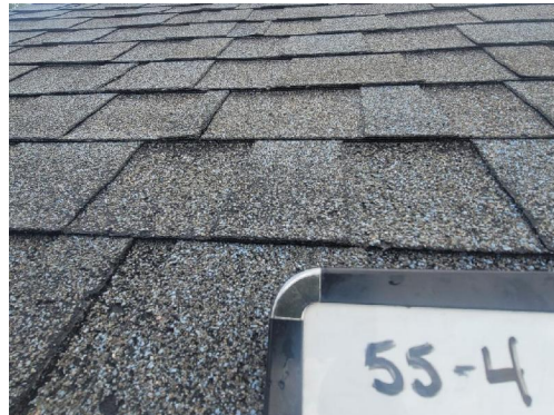
55-4 Asphalt Shingle/Tar Typical Exterior Peaked Roof
