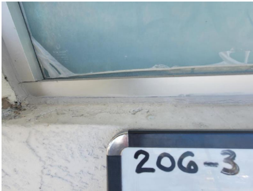
206-3 Caulk Typical Exterior Windows
