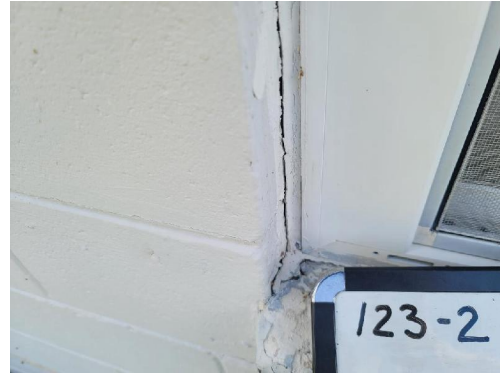
123-2 Caulk Typical Exterior Windows
