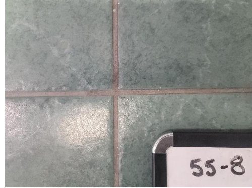
55-8 Grout Typical Interior Hall Tile Flooring
