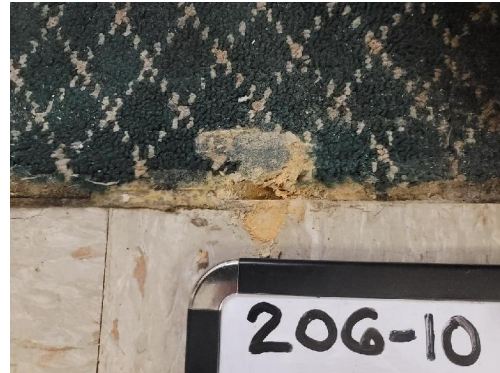
206-10 Carpet Mastic Typical Interior
