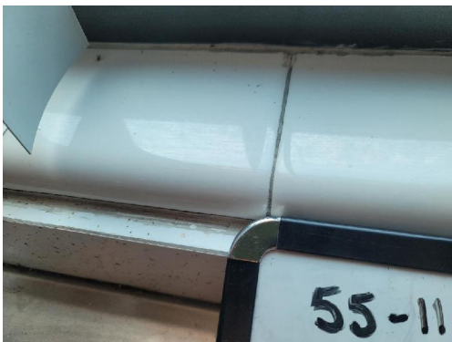
55-11 Grout Typical Interior Window Sill Tile
