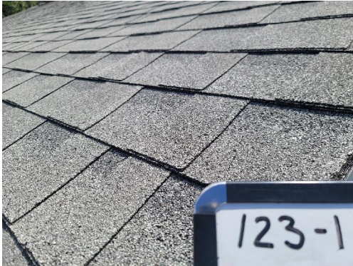
123-1 Asphalt Shingle/Tar Typical Exterior Roof
