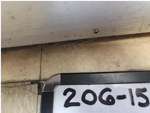
206-15 12"x12" Floor Tile/Adhesive Interior Office
