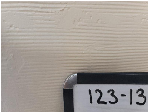
123-13 Wall Tile Mastic Interior Kitchen
