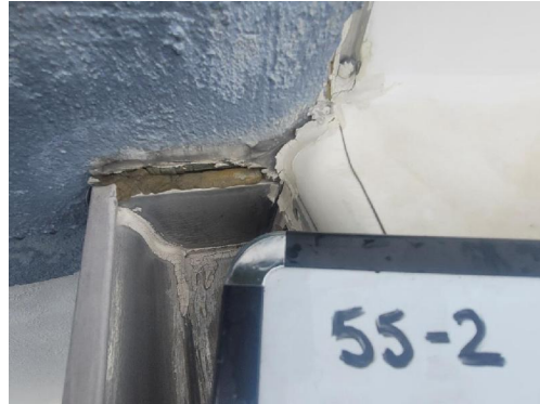
55-2 Caulk Typical Exterior Roof Flashing
