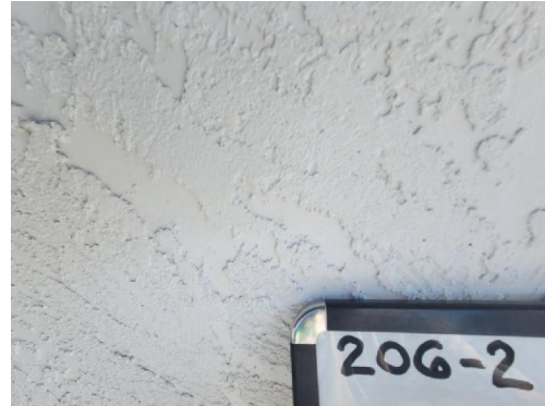
206-2 Stucco Typical Exterior Walls
