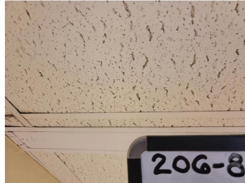
206-8 2'x4' Suspended Ceiling Tile Typical Interior
