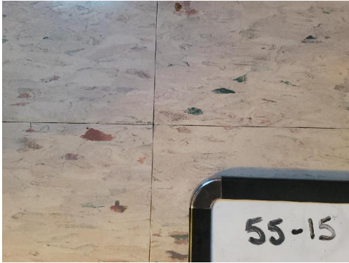
55-15 12"x12" Floor Tile/Mastic Interior North Women's Room
