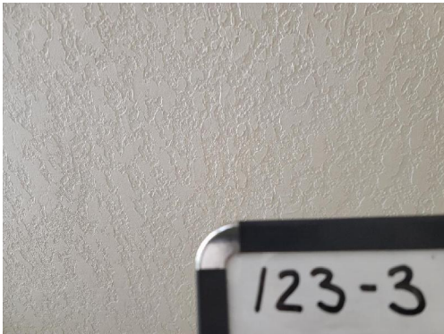
123-3 Drywall/Joint Compound Typical Interior Ceilings
