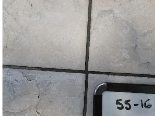
55-16 Grout Interior North Men's Room Tile Flooring
