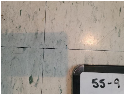
55-9 12"x12" Floor Tile/Mastic Interior Chapel/Kitchen
