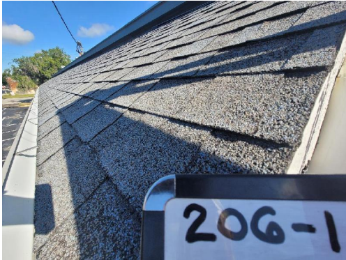
206-1 Asphalt Shingle/Tar Exterior Roof Overhangs
