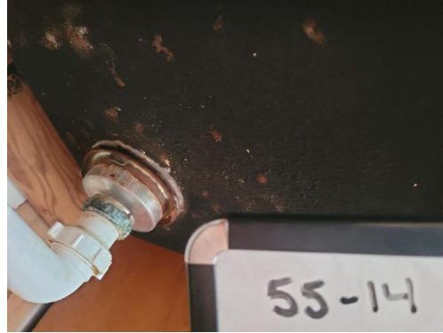
55-14 Sink Mastic/Black Interior Kitchen 4% Chrysotile
