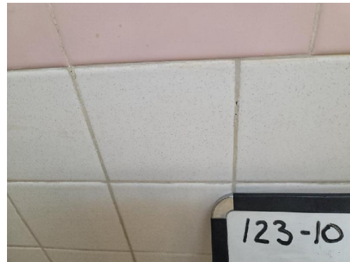
123-10 Grout Interior Bathroom Wall Tile
