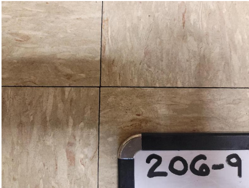
206-9 12"x12" Floor Tile/Adhesive Typical Interior Main/Top Layer
