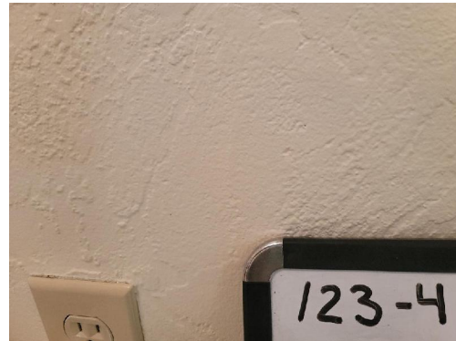
123-4 Plaster Typical Interior Walls
