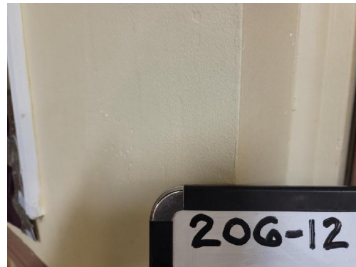
206-12 Drywall/Joint Compound Typical Interior Walls
