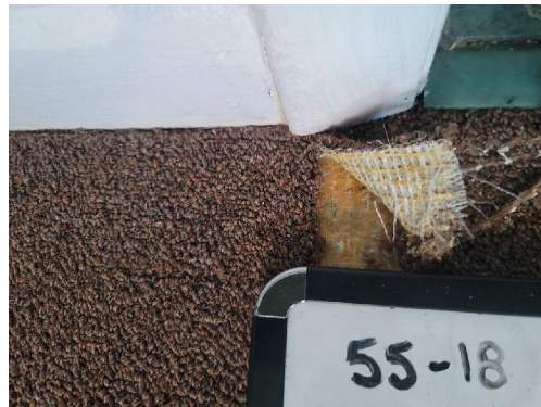
55-18 Carpet Mastic Typical Interior
