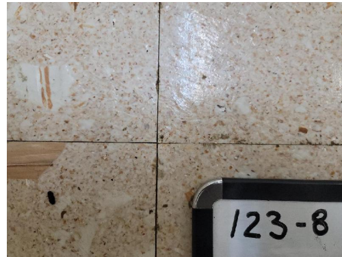
123-8 12"x12" Floor Tile/Adhesive Interior Bathroom
