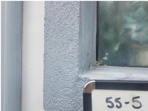
55-5 Caulk Typical Exterior Windows/Doors
