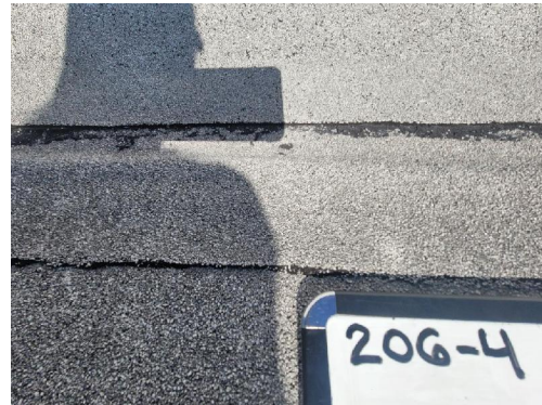
206-4 Rolled Asphalt Roofing/Tar Typical Exterior Main Roof
