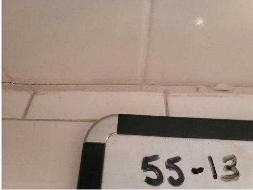
55-13 Caulk Interior Baptismal Pool Tile
