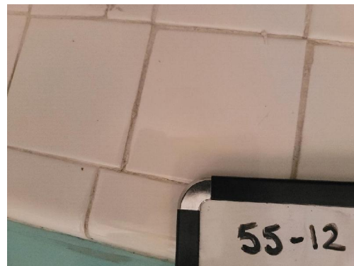
55-12 Grout Interior Baptismal Pool Tile
