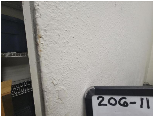
206-11 Plaster Typical Interior Walls/Ceilings
