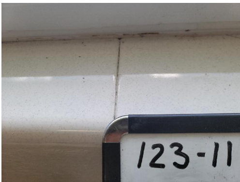
123-11 Grout Typical Interior Tile Window Sills
