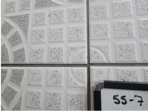
55-7 Grout Interior Front Entry Tile Flooring
