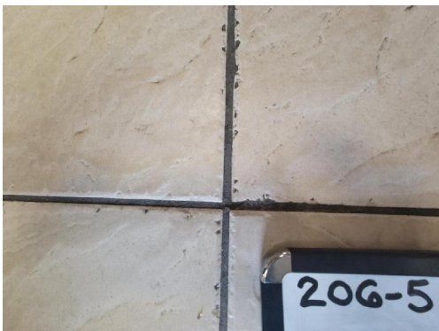
206-5 Grout Interior Rear Entry Tile Flooring
