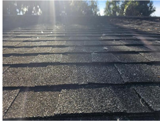
1928-4 Asphalt Shingle/Tar Typical Exterior Roof
