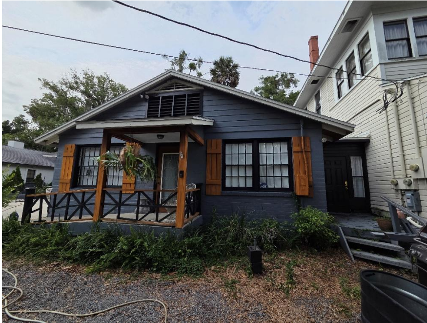
Existing Condition – Attached building.
