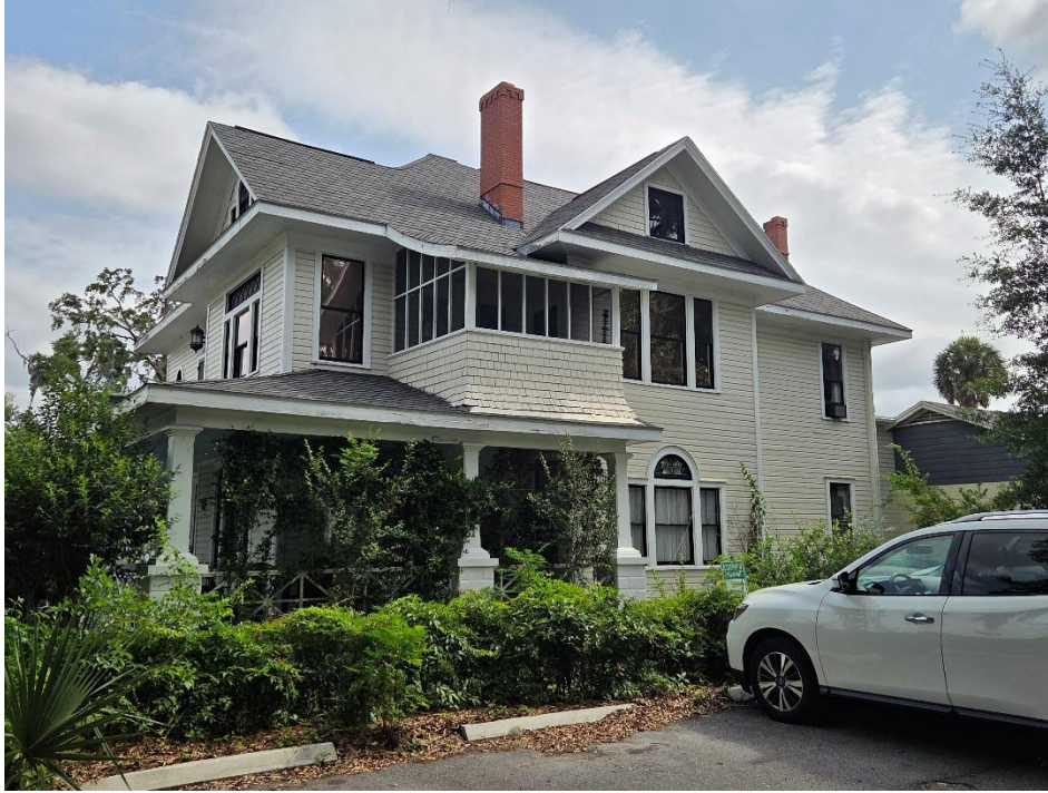
Existing Condition of façade.
