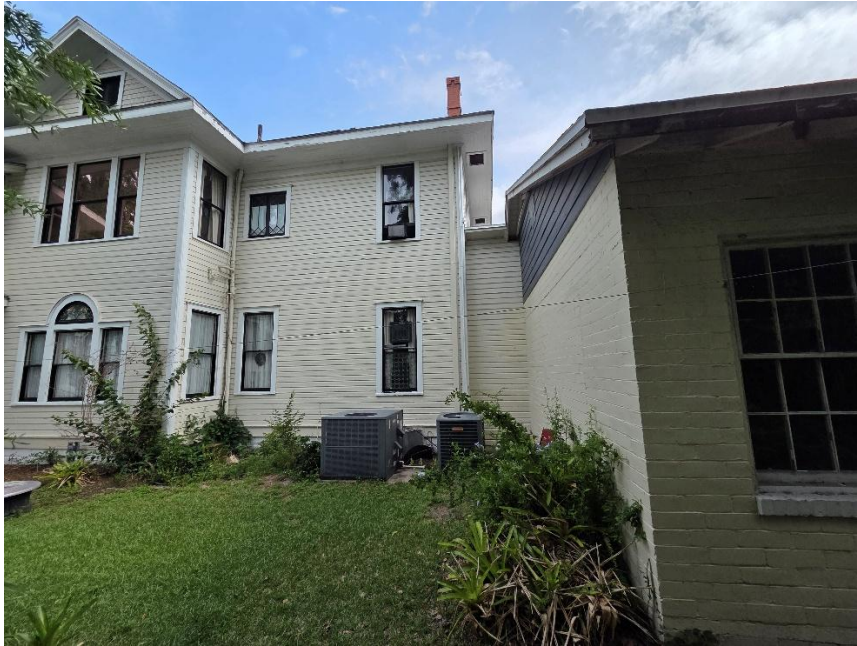
Existing condition – exterior
