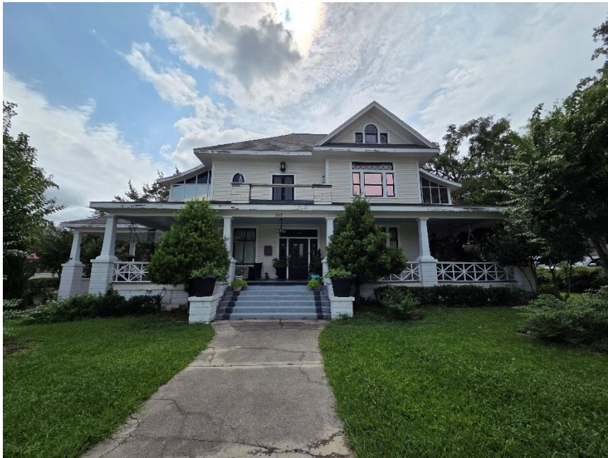
Existing condition – exterior
