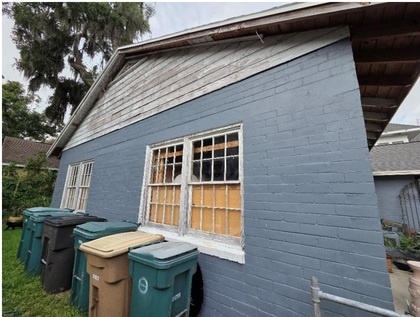
Existing condition of attached building – exterior
