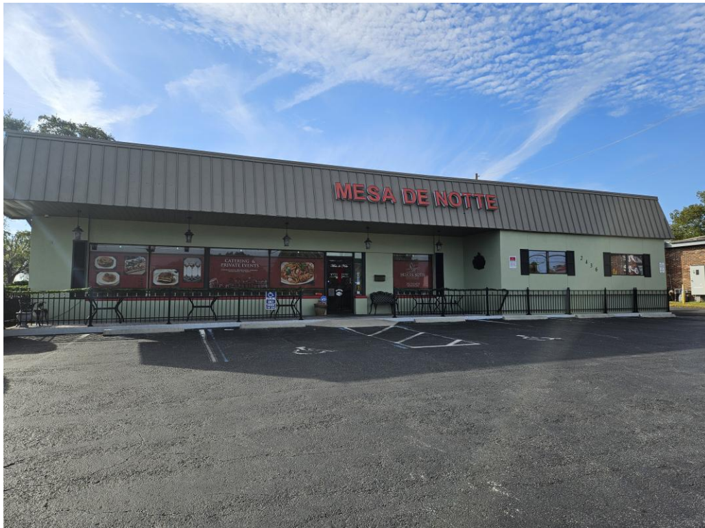
Image 1- Existing conditions -Front view from Silver Springs Blvd.
