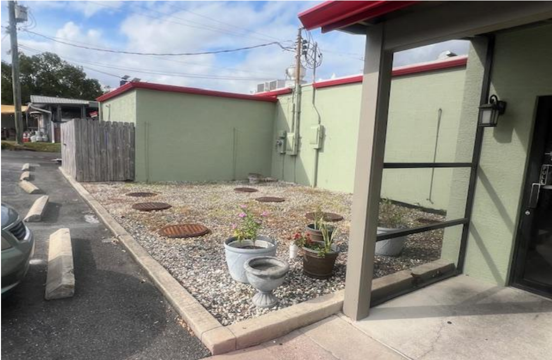
Image 5 -Existing condition – Rear view and entrance
