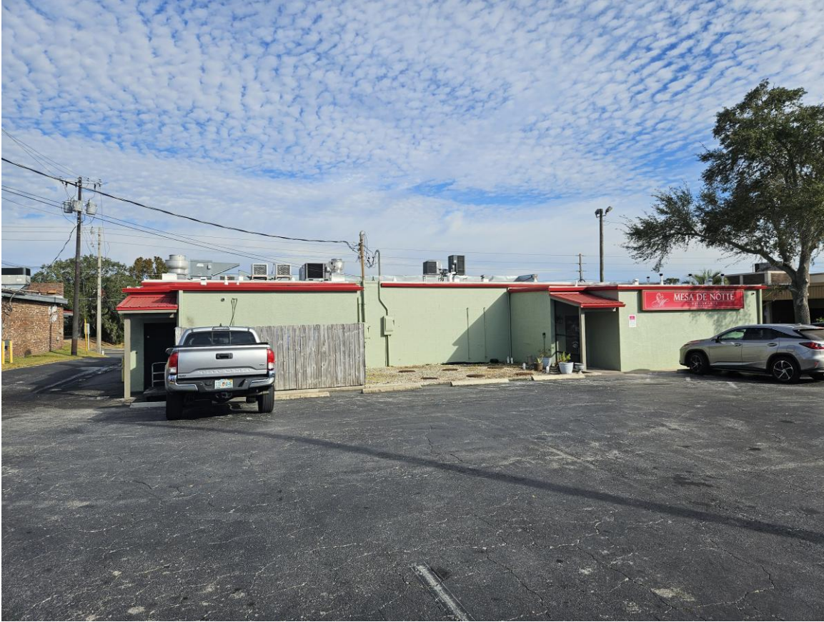
Image 6 – Existing condition of parking lot
