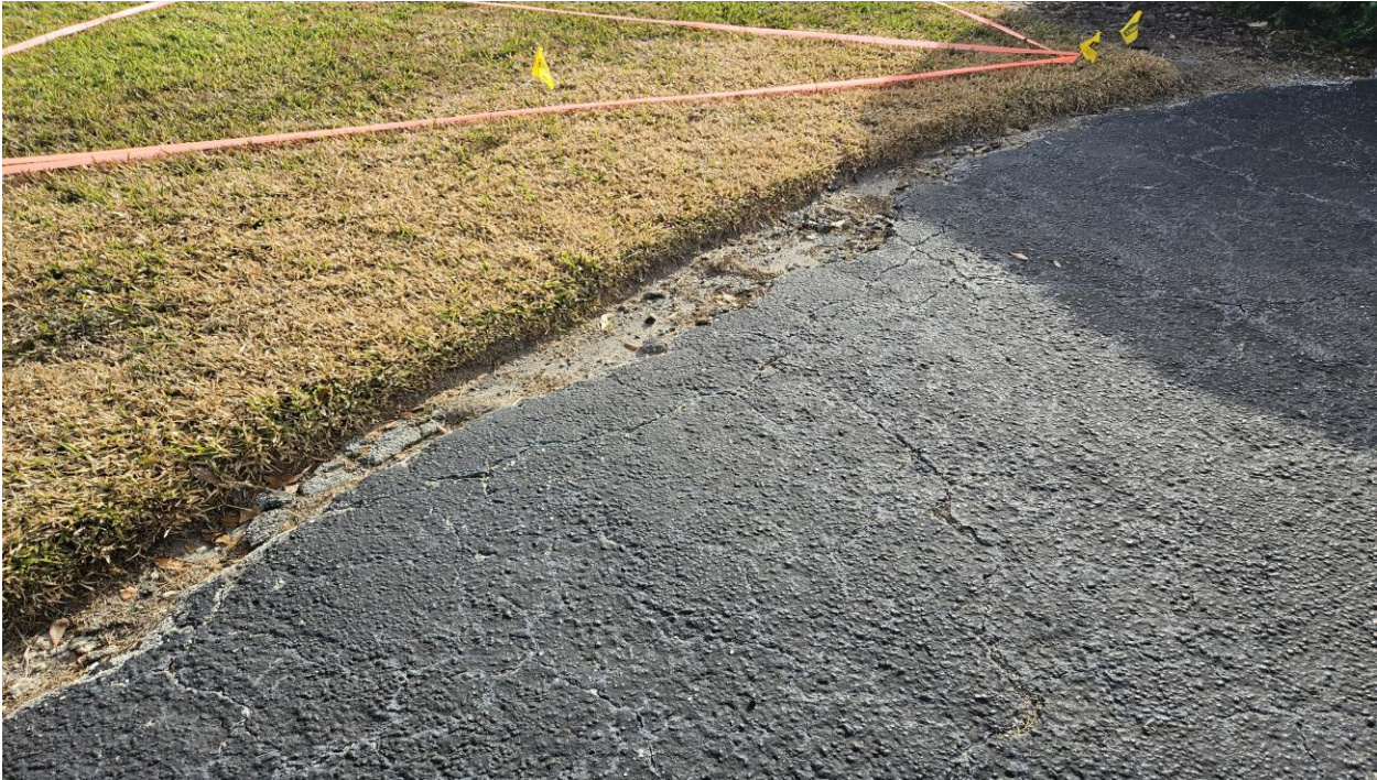
Image 8. Existing condition of parking lot
