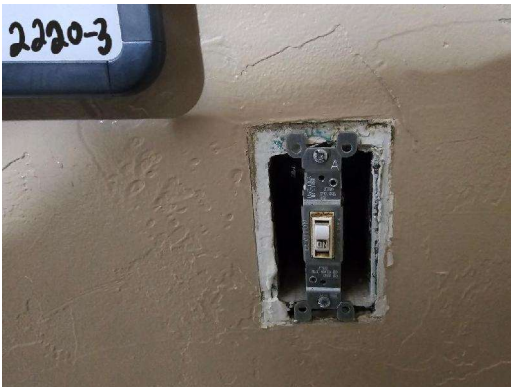
2220-3 Joint Compound (2% Chrysotile) Drywall Typical Interior Walls/Ceilings
