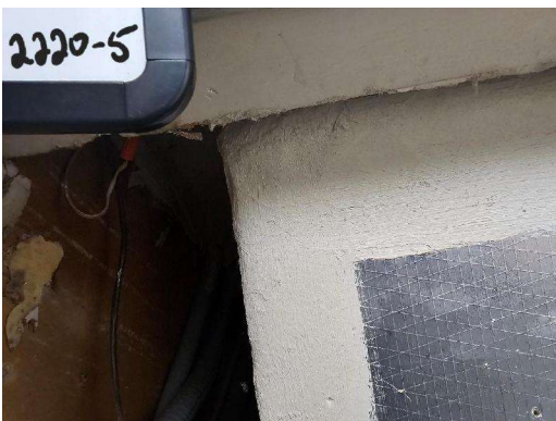
2220-5 Duct Mastic Typical Interior HVAC
