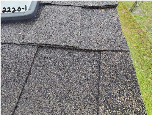
2220-1 Asphalt Shingle/Tar Typical Exterior Roof
