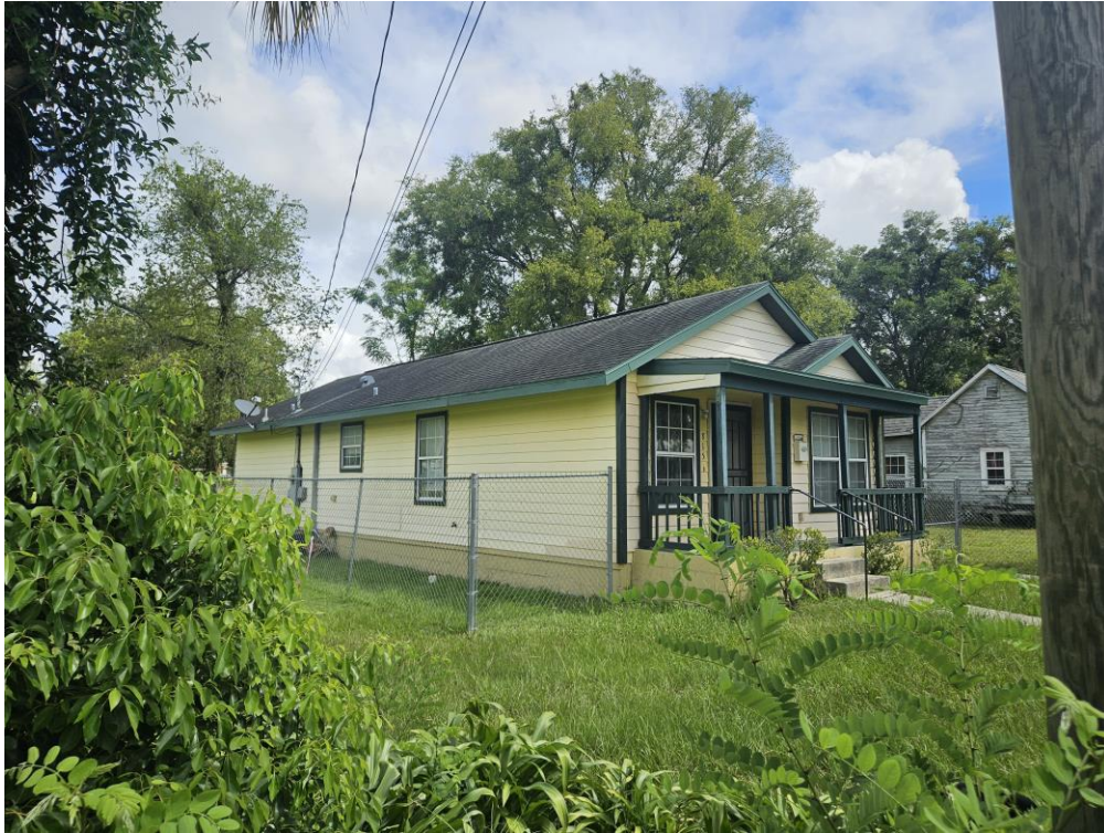
Image 1. View of the roof looking Northeast from West Silver Springs Place.
