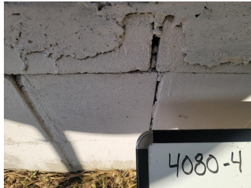
4080-4 Concrete Block/Mortar Exterior Front Porch
