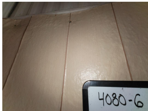
4080-6 Paneling South Enclosed Porch Walls
