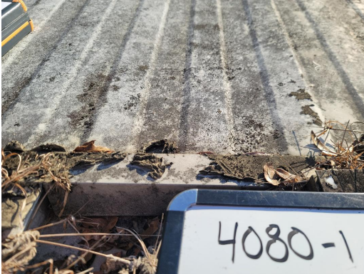
4080-1 Roof Coating Typical Exterior Roof
