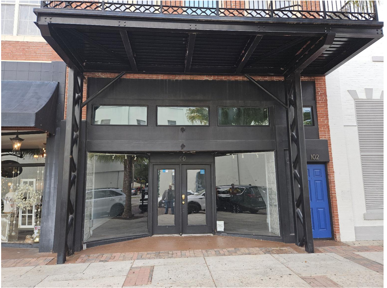
Existing store façade.
