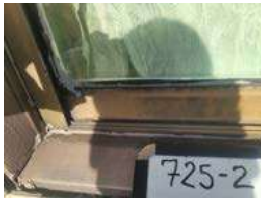
725-2 Caulk Typical Exterior Windows
