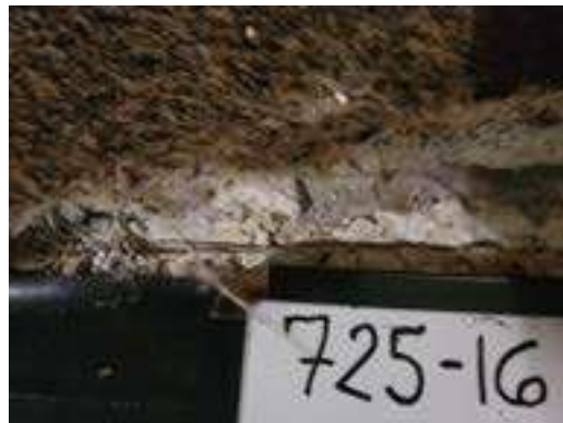
725-16 Floor Leveling Compound Interior NE Bedroom
