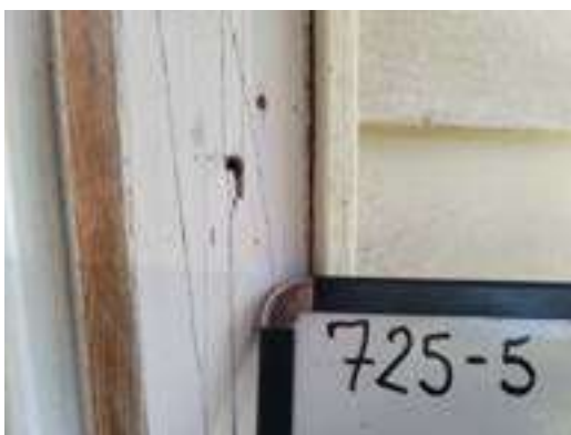
725-5 Caulk Exterior Front Door
