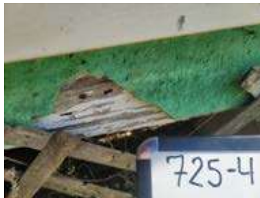
725-4 House Wrap Typical Exterior Walls
