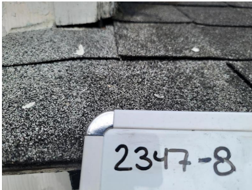
2347-8 Asphalt Shingle Typical Exterior Roof
