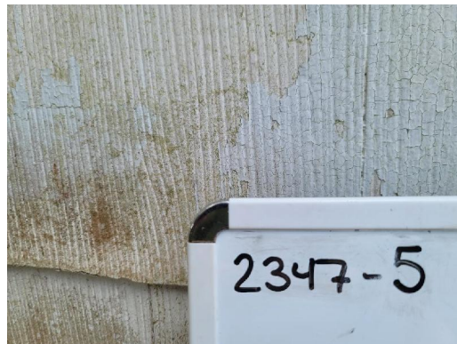
2347-5 Transite Siding (10% Chrysotile) Typical Exterior Walls
