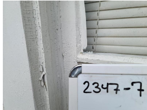
2347-7 Window Glazing (<1% Chrysotile) 5 Exterior Windows
