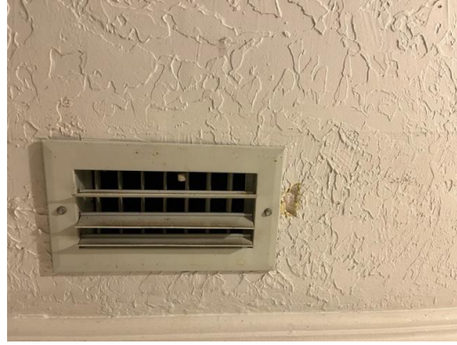
901-2 Texture Joint Compound/Yellow (6% Chrysotile) Drywall Typical Interior Walls/Ceilings
