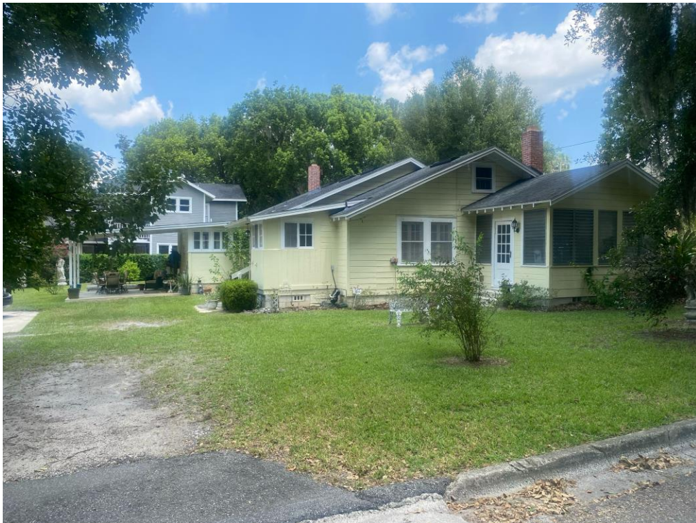
South elevation facing north on SE 6 th Street.
