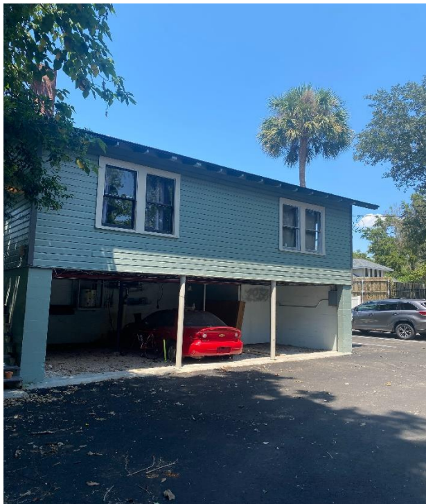
In the rear yard of 709 E Fort King Street, facing north viewing the existing accessory structure.
