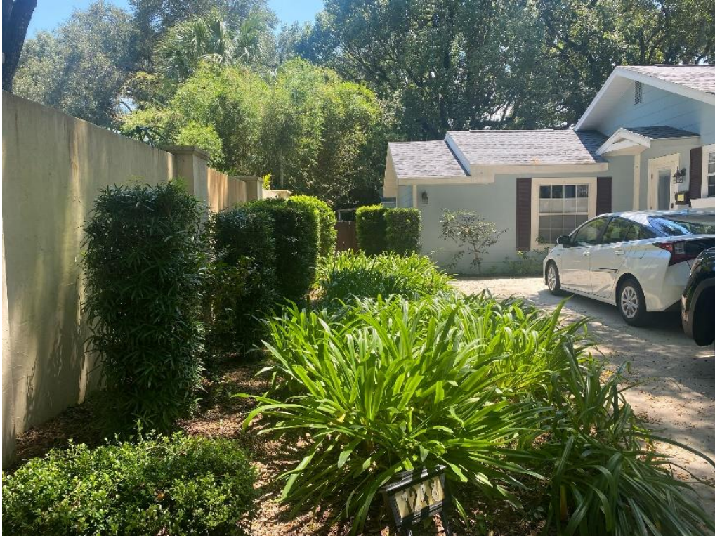
Eastern side yard and view of wooden gate to be replaced, facing south onto subject property.
