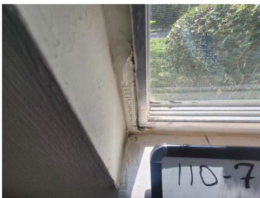
110-7 Caulk/Wrap/Adhesive Typical Interior Windows
