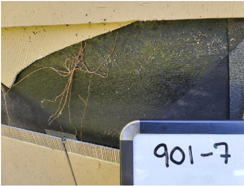
901-7 Felt House Wrap Typical Exterior Walls
