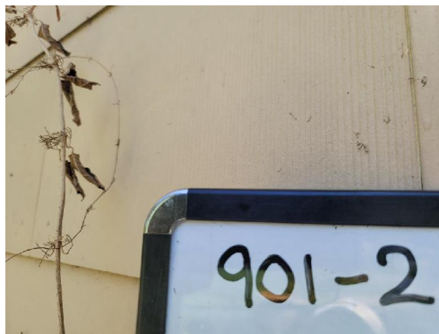
901-2 Transite Siding/Gray (15% Chrysotile) Typical Exterior Walls
