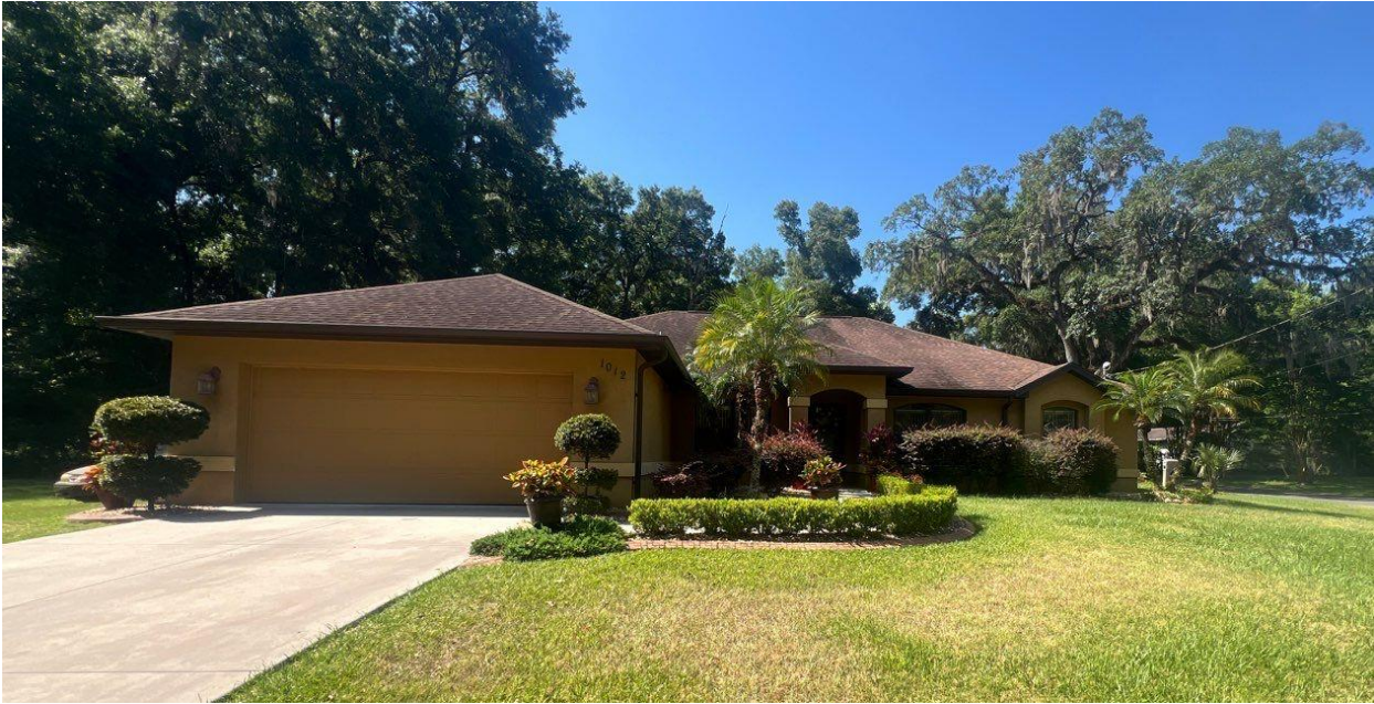
Existing condition - painting
