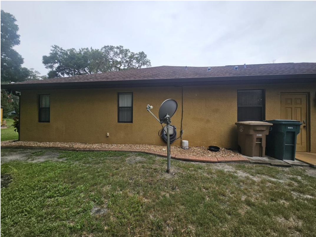
Existing condition - painting
