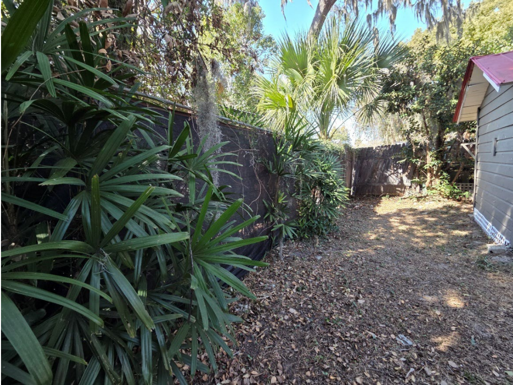
Prep Work and Fence (continued)
