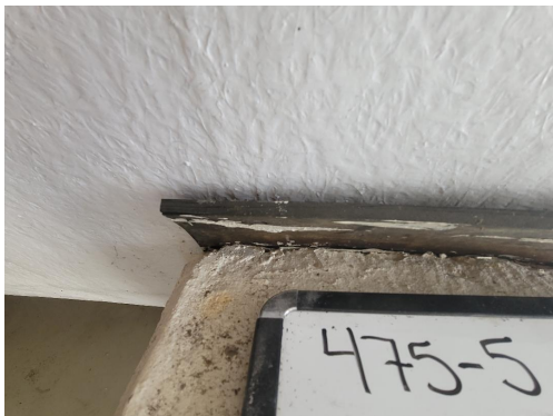
475-5 Padding/Black Typical Interior Tank Supports
