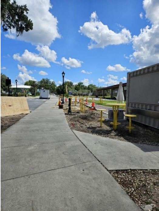
DOWNTOWN MARKET - IMPROVEMENTS IN-PROGRESS
