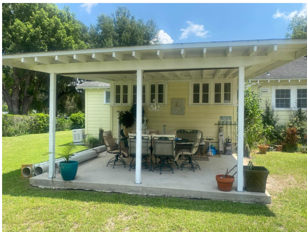
The west and south elevation of porch and existing columns.
