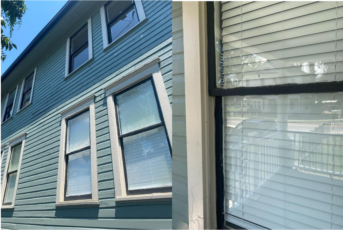
The current windows to be replaced.
