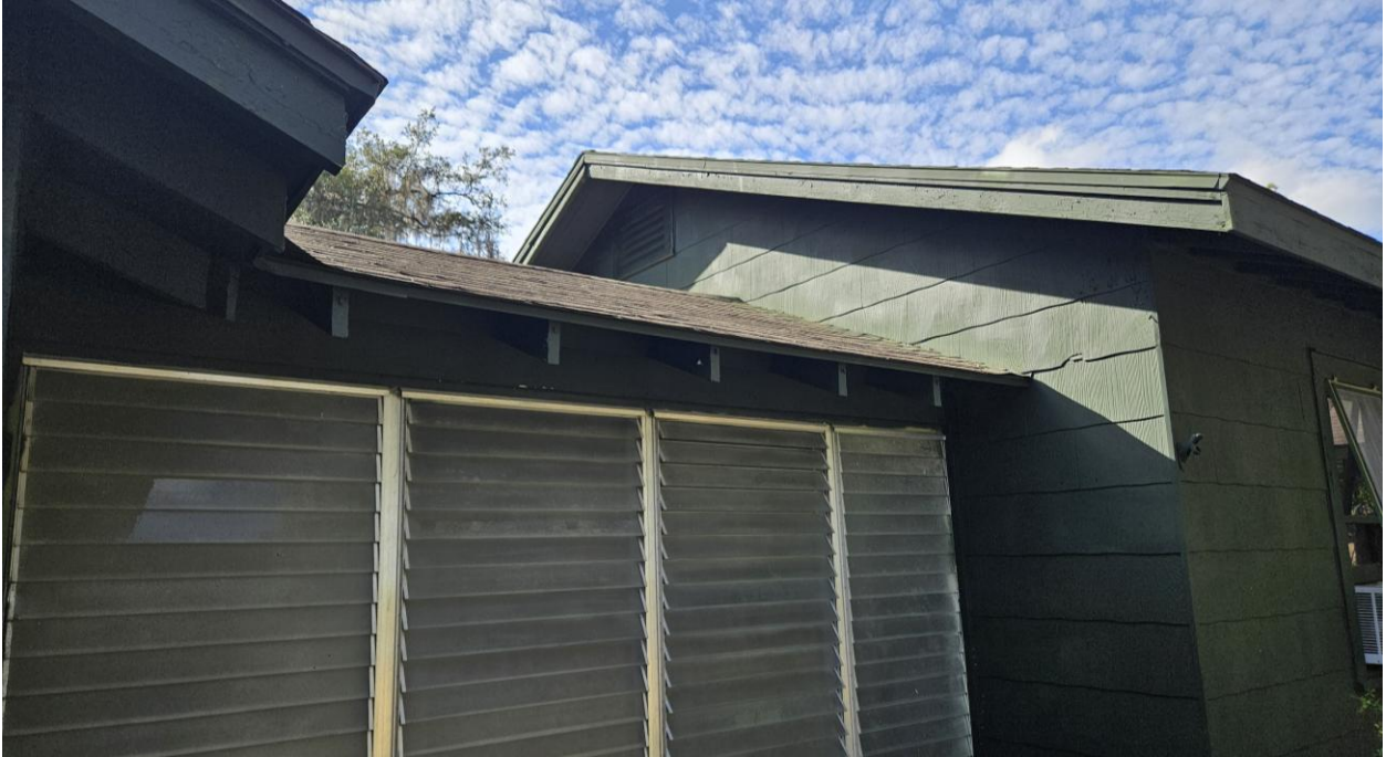
Image 2 Existing roof condition
