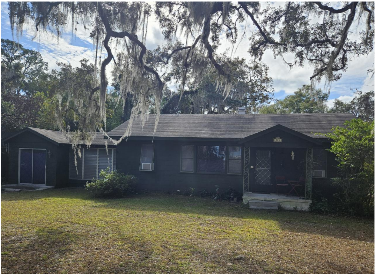
Image 1- Existing roof condition
