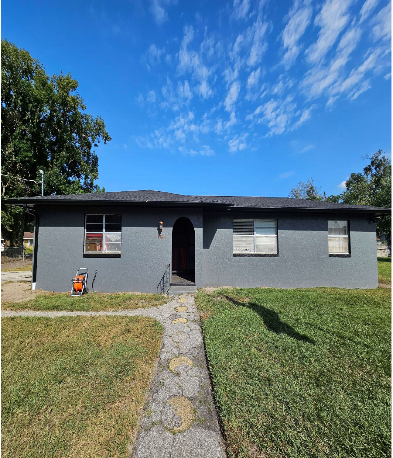
Image 1 Front view of the property
