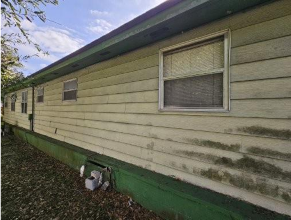
Image 3 – Existing conditions of windows and building façade.
