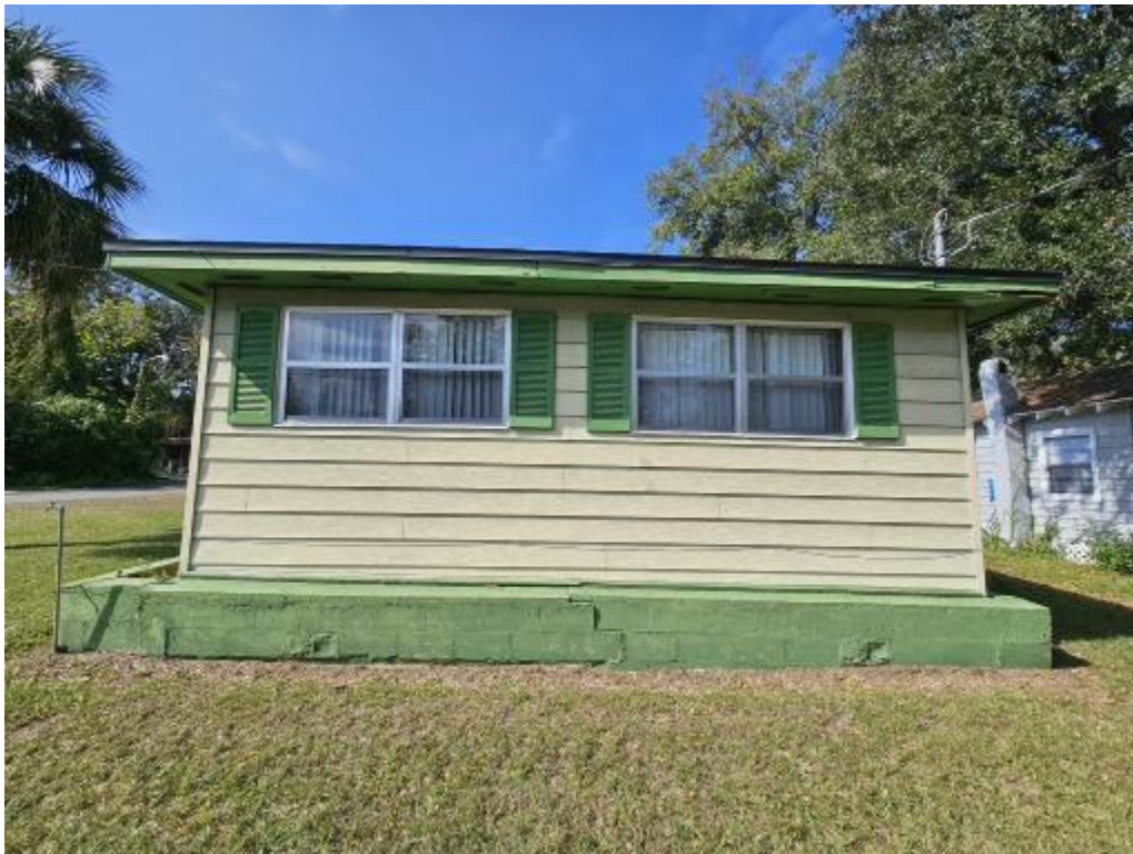
Image 2- Existing conditions of windows and building façade.
