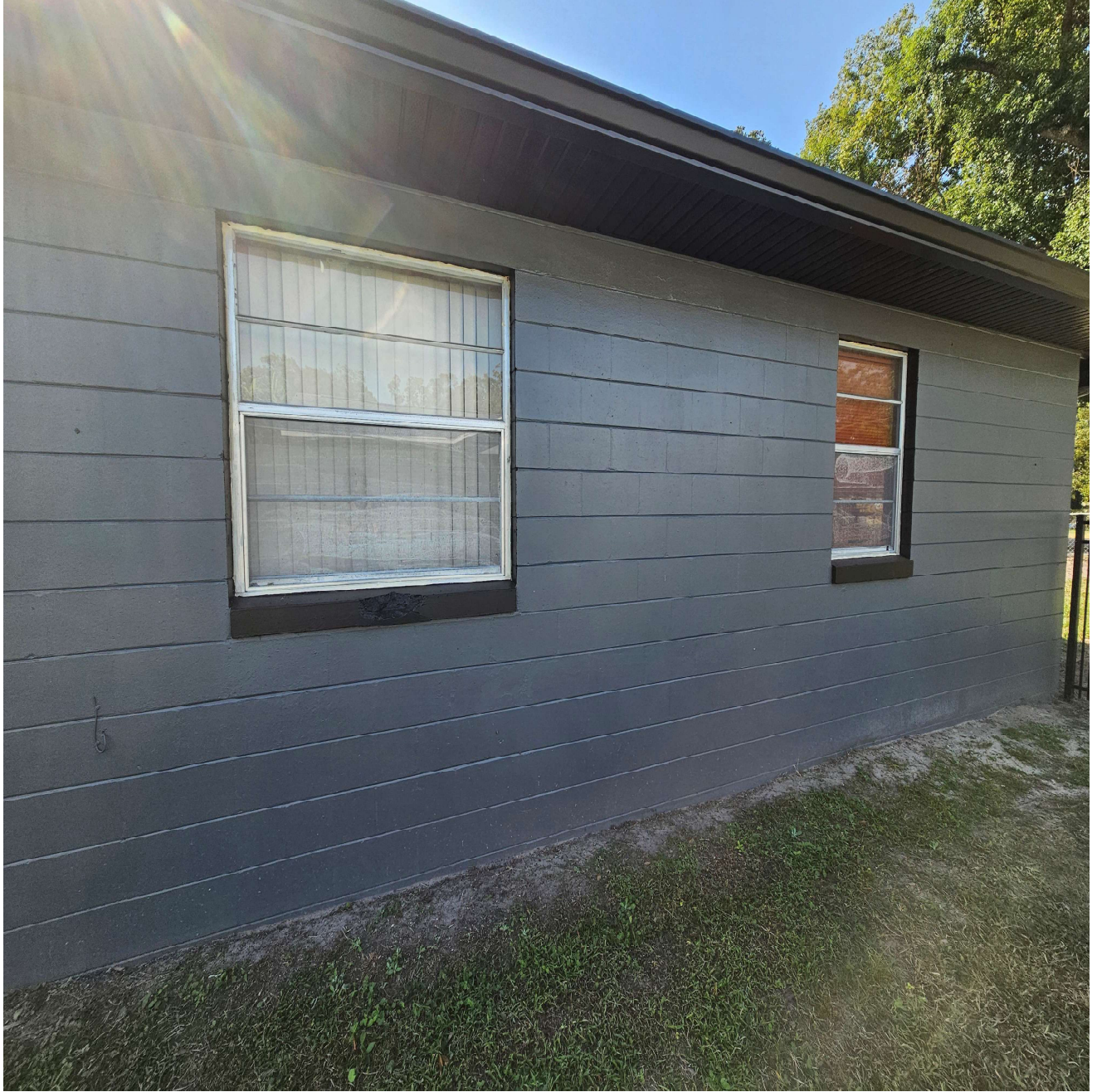
Image 3 View of existing window.
