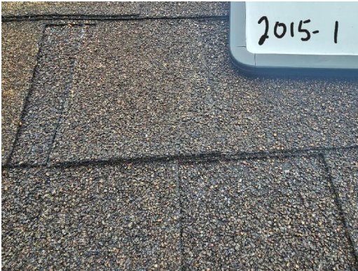
2015-1 Asphalt Shingle/Tar Typical Exterior Roof
