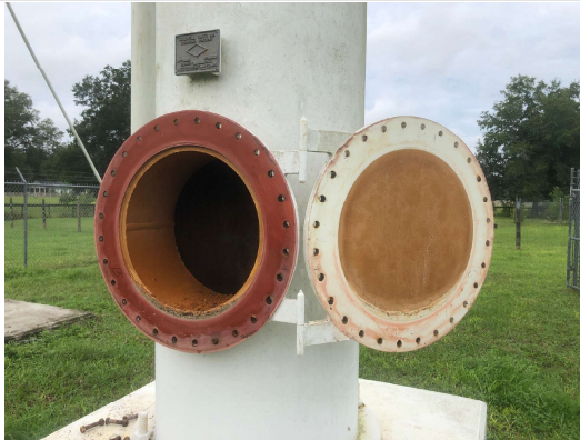
Interior base of wet riser / outlet
