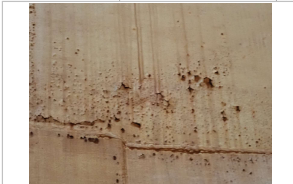
Internal walls (corrosion / d-lamination)
