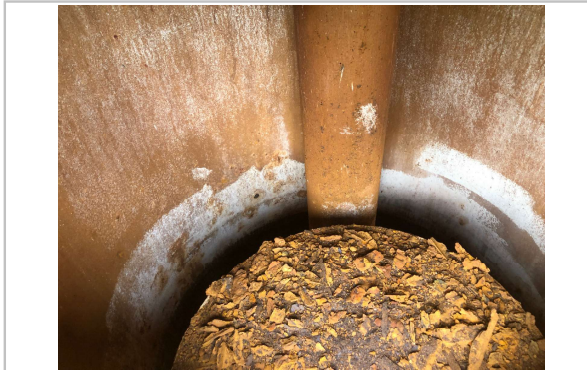
Internal walls (corrosion / d-lamination)
