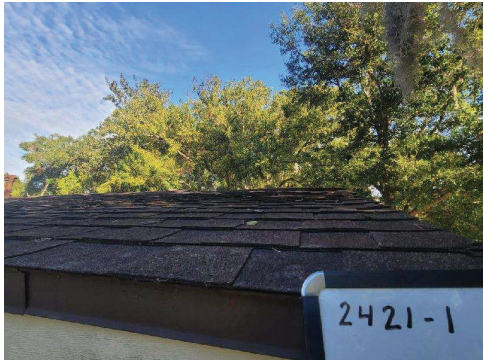
2421-1 Asphalt Shingle Typical Exterior Roof
