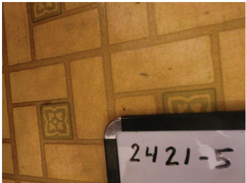
2421-5 Rolled Flooring/Tan (15% Chrysotile) Adhesive Interior Hall Bathroom (Appx 20 sq ft)
