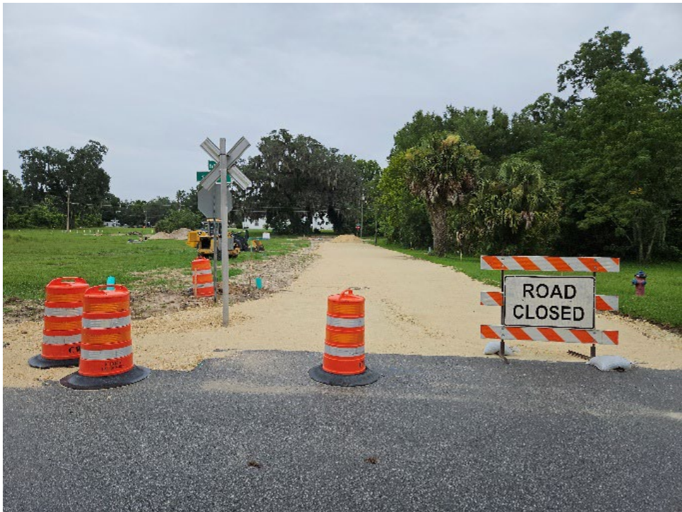
Figure 13. Road construction in progress.
