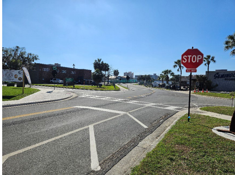
Figure 27. Improvements at the intersection of NE Watula Avenue and NE 3 rd Street.
