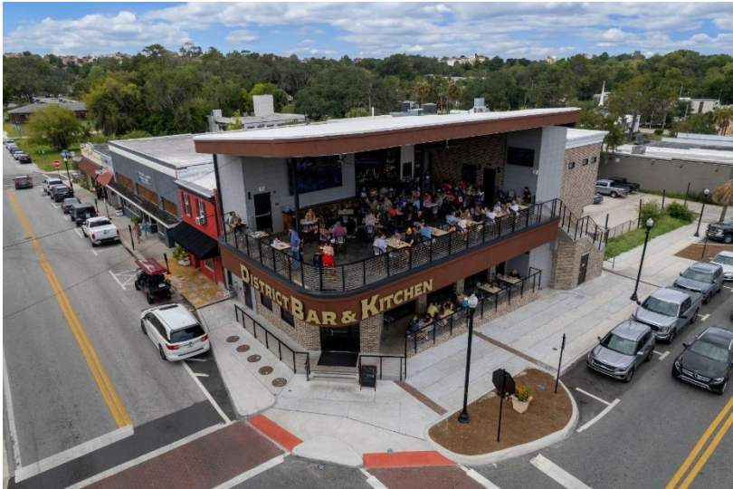
Figure 65. After – project completion. Photo credits: Maven Photo & Film and District Bar & Kitchen
