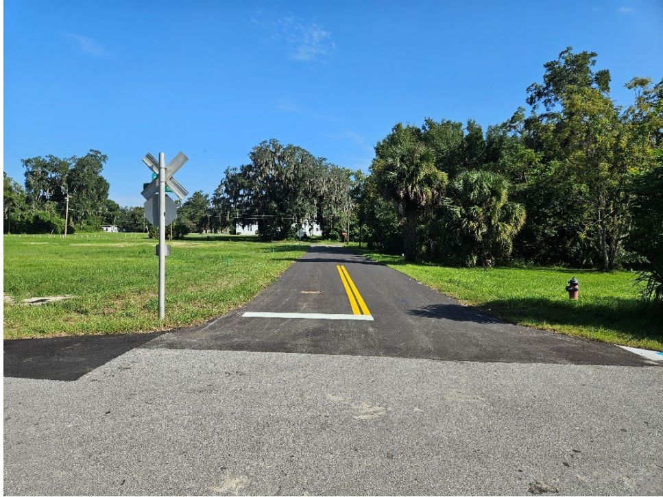
Figure 14. Newly constructed road.
