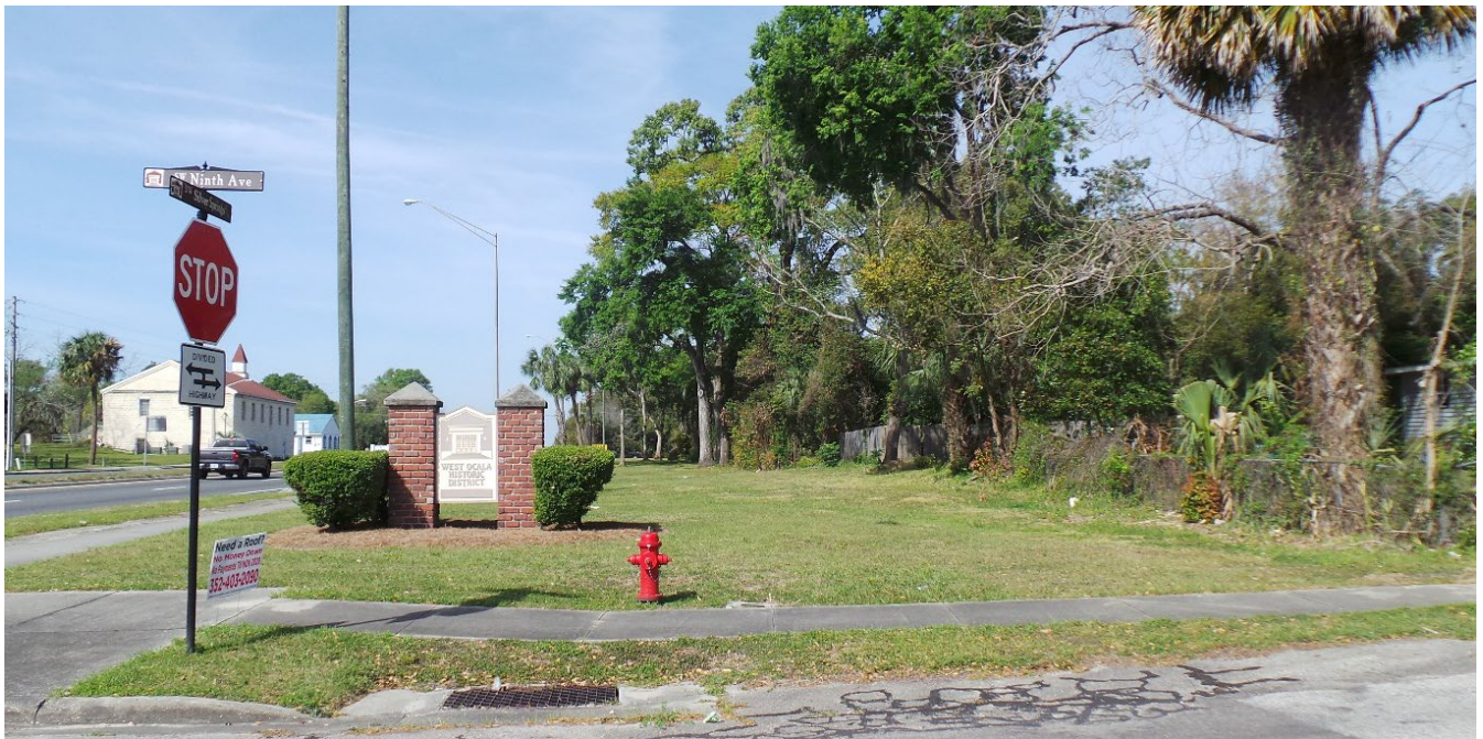
Figure 3. Site conditions before improvements, looking west along West Silver Springs Boulevard.
