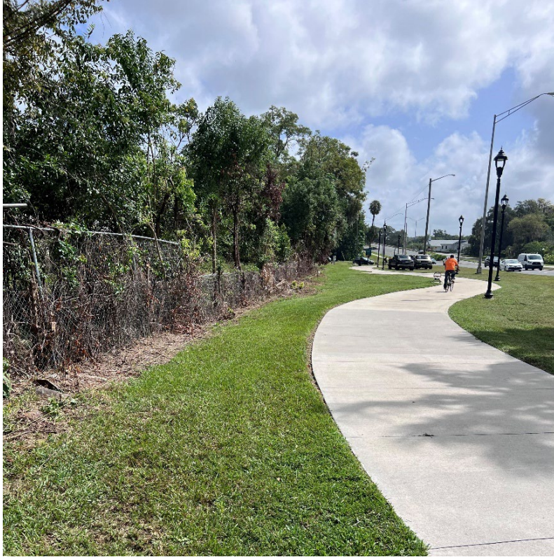
Figure 7. Property line before fence installation.
