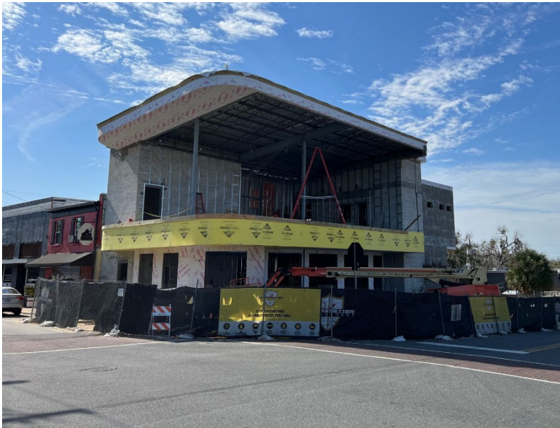
Figure 63. Construction - in progress.
