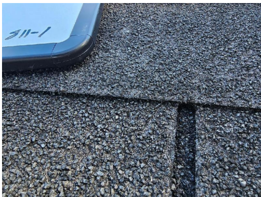
811-1 Asphalt Shingle/Tar Typical Exterior Roof
