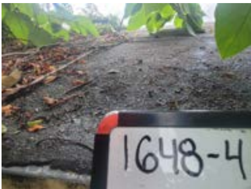
1648-4 Rolled Asphalt Roofing Typical Exterior Shed Roof
