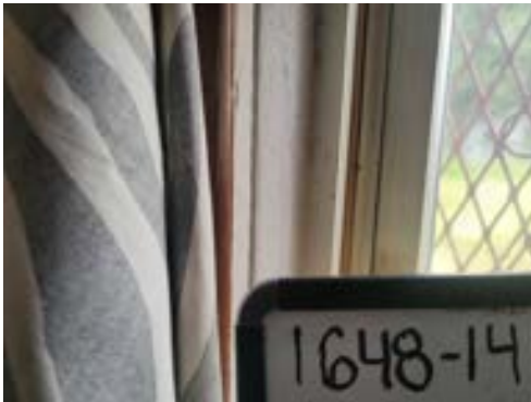
1648-14 Caulk Typical Interior Windows
