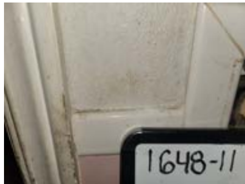
1648-11 Ceramic Tile/Grout Typical Interior Bathroom Walls
