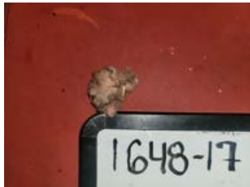
1648-17 Insulation Typical Interior
