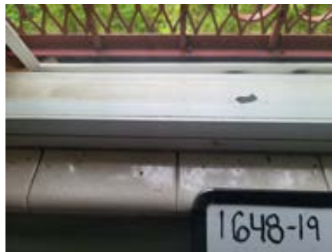
1648-19 Ceramic Tile/Grout Typical Interior Window Sills
