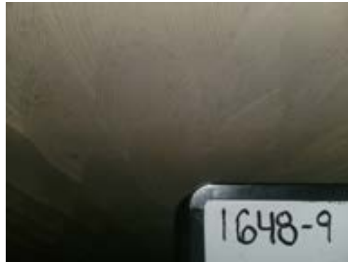
1648-9 Drywall/Joint Compound Typical Interior Walls/Ceilings
