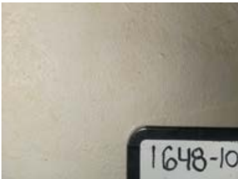
1648-10 Plaster Typical Interior Walls/Ceilings
