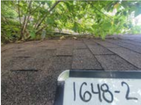
1648-2 Asphalt Shingle/Tar Typical Exterior House Roof
