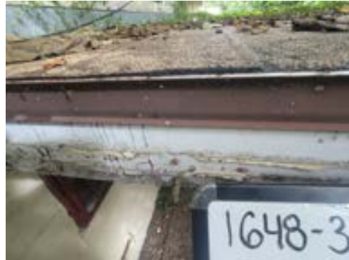
1648-3 Caulk Typical Exterior Flashing
