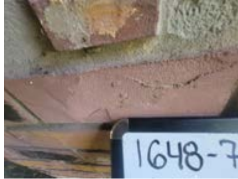
1648-7 Brick/Mortar Exterior Front Porch Walls
