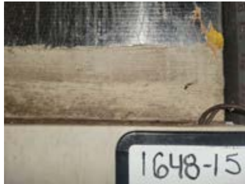
1648-15 Duct Mastic Typical Interior HVAC
