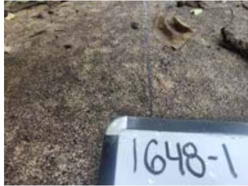
1648-1 Rolled Asphalt Roofing Typical Exterior House Roof
