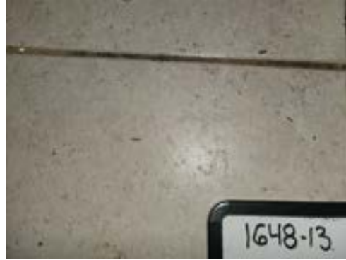
1648-13 2'x2' Ceramic Tile/Grout Typical Interior Floors
