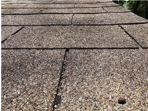
2612-1 Asphalt Shingle/Tar Typical Exterior Roof
