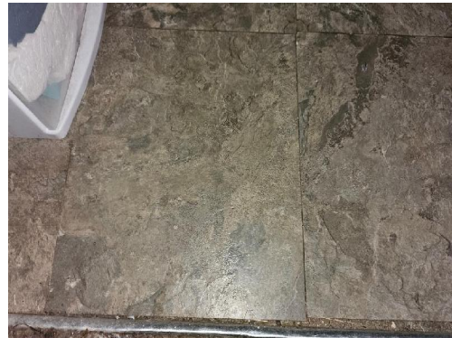
2612-4 12"x12" Floor Tile/Adhesive Typical Interior Bathrooms
