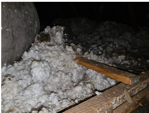
2612-5 Insulation Typical Interior
