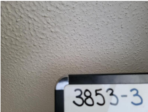
3853-3 Popcorn Ceiling Texture Interior HVAC Closet
