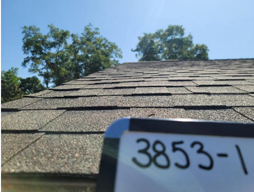
3853-1 Asphalt Shingle/Tar Typical Exterior Roof
