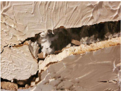
1635-5 Insulation Typical Interior
