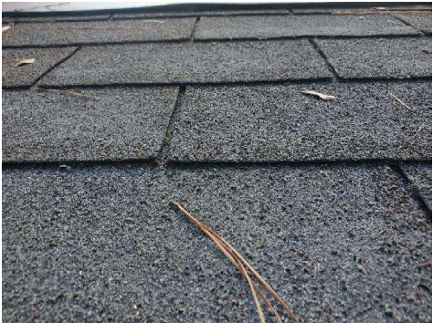
1635-1 Asphalt Shingle/Tar Typical Exterior Roof
