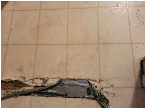
1635-2 Rolled Flooring/Mastic Living Room/Bedrooms
