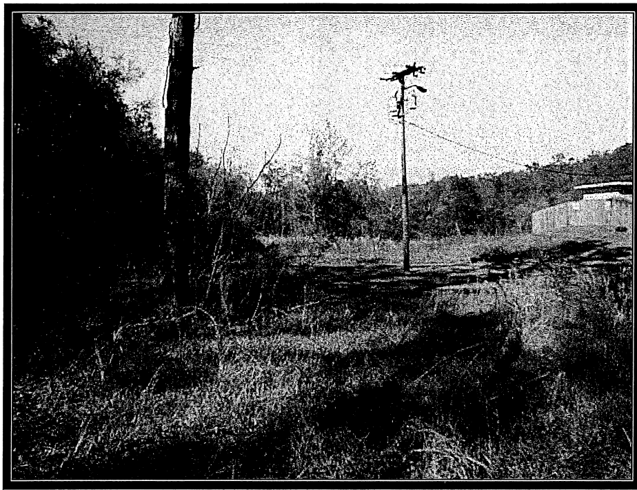
View of low lying area between NW 16 th Avenue and radio tower pad site
