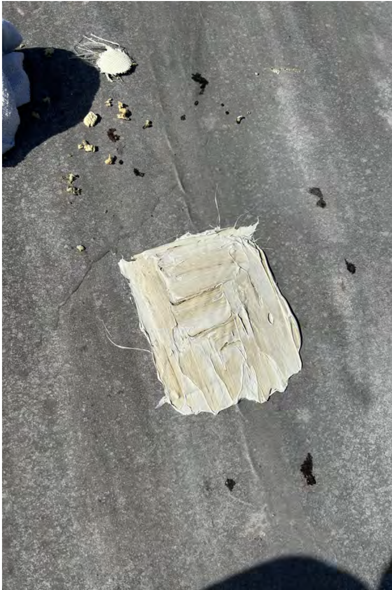
Core Cut Repair
