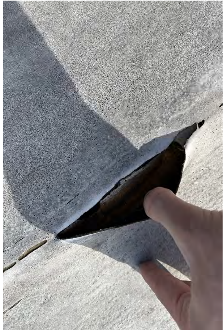
Hole in Membrane
