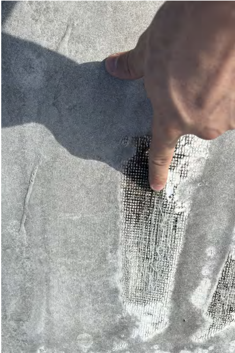
Hole in Membrane
