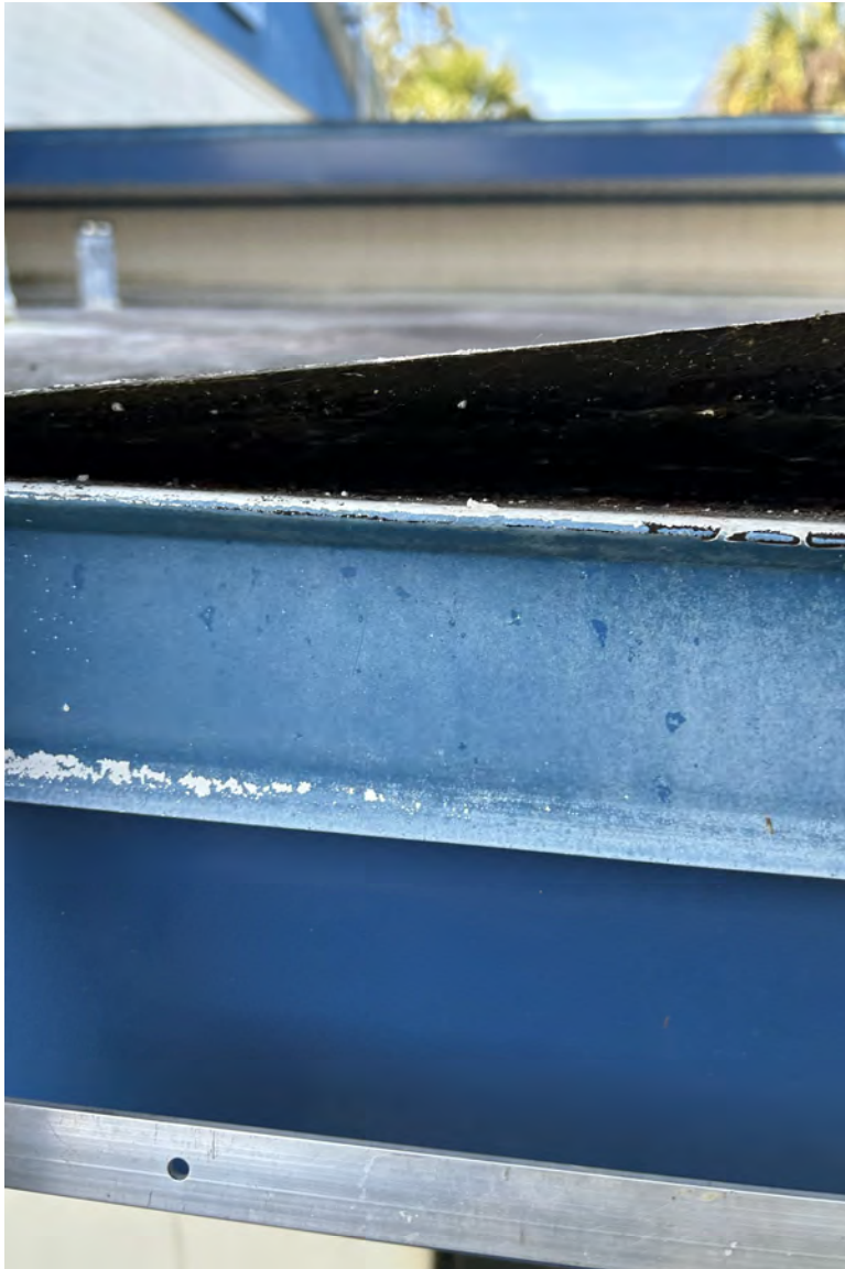
Cap Sheet not Adhered to Metal Perimeter
