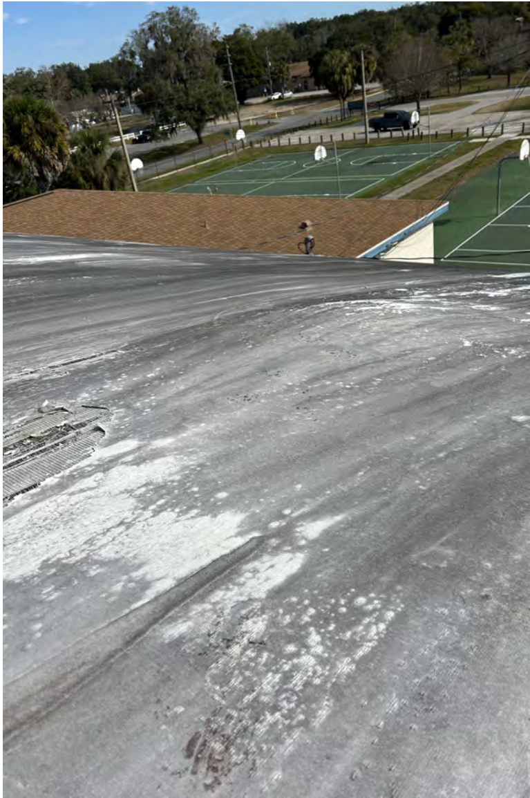
Holes in Membrane
