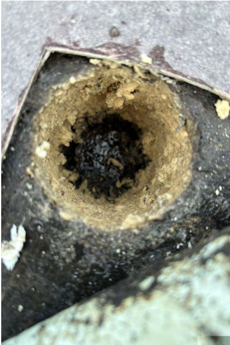
Core Cut Showing Wet Deck
