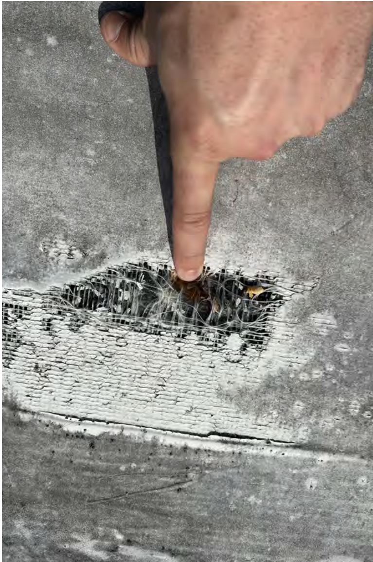
Hole in Membrane
