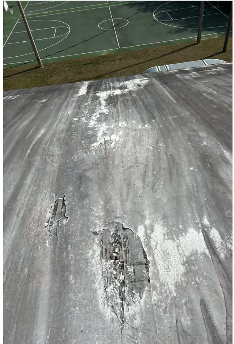
Holes in Membrane
