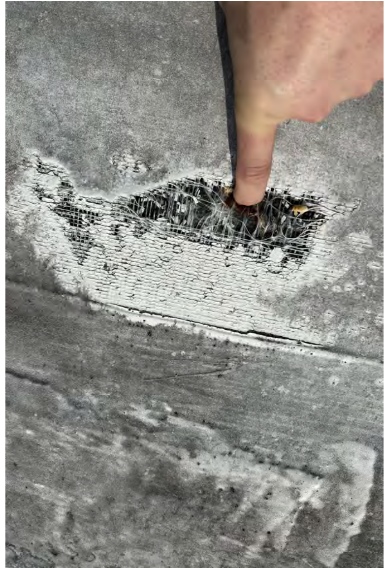
Hole in Membrane
