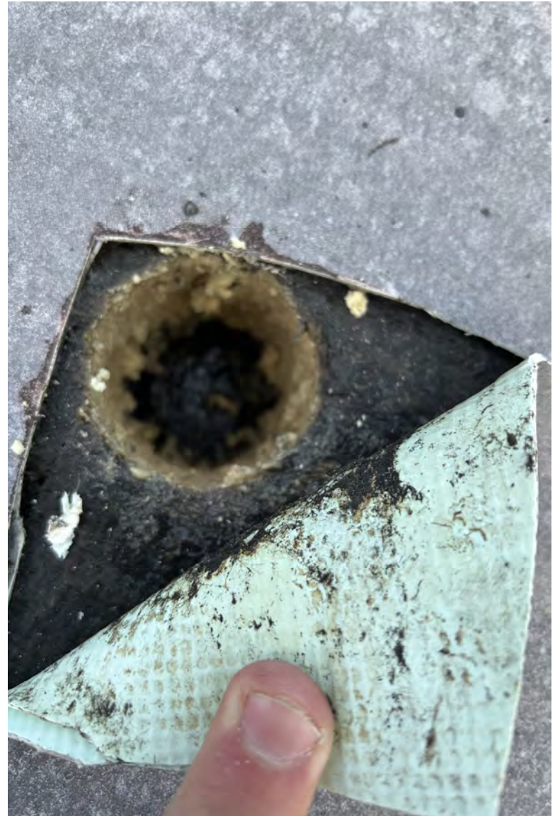
Core Cut Showing Wet Deck
