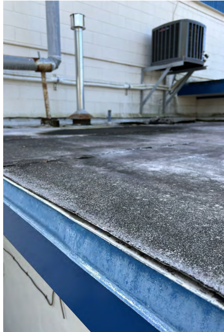
Cap Sheet not Adhered to Metal Perimeter
