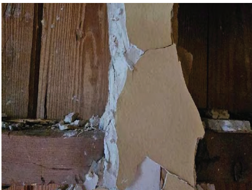
719-1 Drywall/Joint Compound Typical Interior Walls/Ceilings
