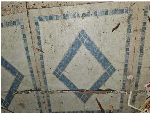
719-3 12"x12" Floor Tile/Mastic Interior Bathroom/Hallway
