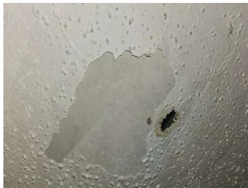
719-2 Surfacing Material Typical Interior Ceilings
