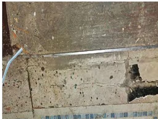
719-4 12"x12" Floor Tile/Gray (2% Chrysotile) Mastic Interior Hallway (Appx 15 sq ft)
