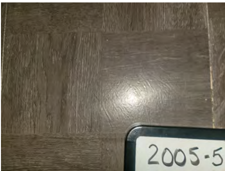
2005-5 12"x12" Vinyl Floor Tile/Adhesive Interior SW Bedroom
