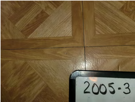
2005-3 12"x12" Vinyl Floor Tile/Adhesive Interior Living Room
