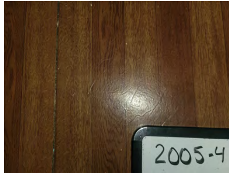
2005-4 12"x12" Vinyl Floor Tile/Adhesive Interior NW Bedroom, NE Bedroom
